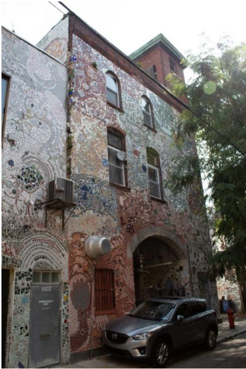
Figure 7 South elevation, 1016-18 South Street. (Source: Author, 2020)
