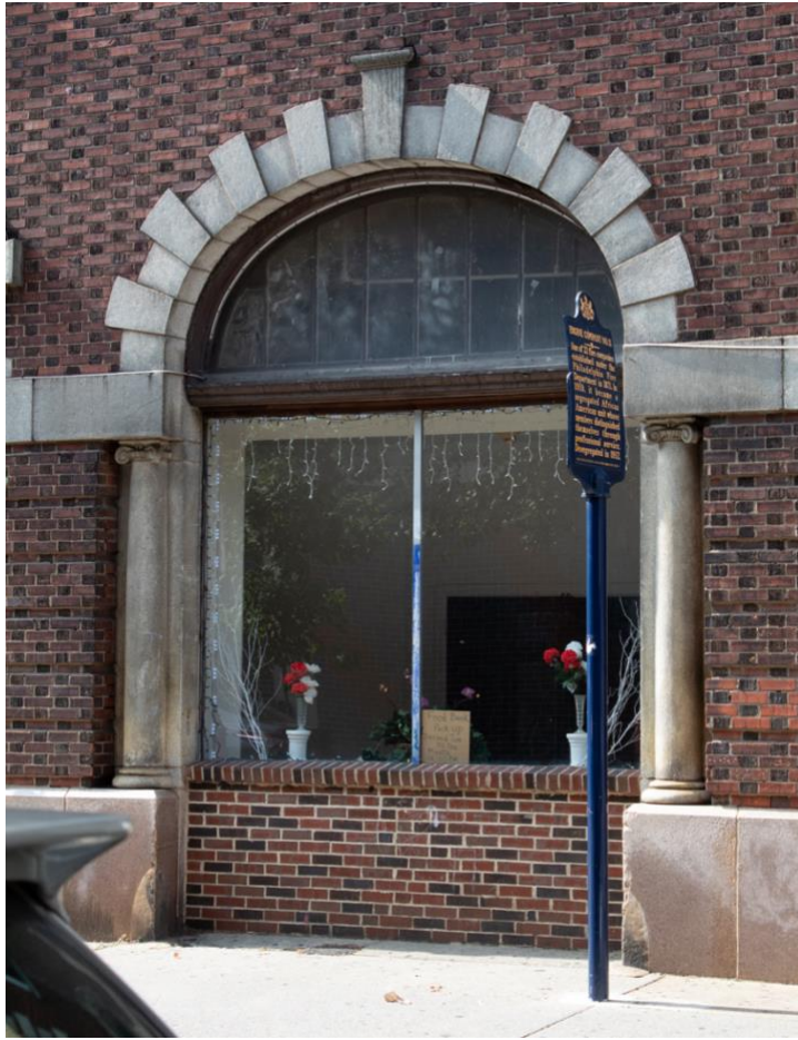
Figure 4 Detail, engine door, 1016-18 South Street. (Source: Author, 2020)
