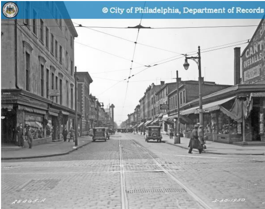
Figure 13 South Street looking west from 10th Street, April 1930. Note Engine 11 with granite quoining at left center. (Source: PhillyHistory.org)
