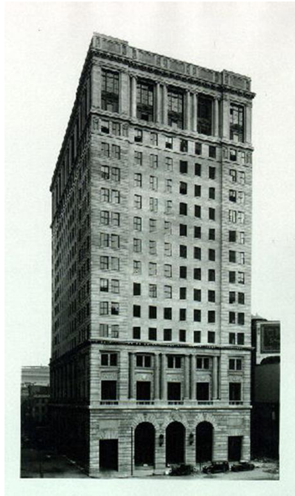
Figure 23 City Hall Annex, 23-31 N Juniper St. (Source: Philadelphia Architects and Buildings )
