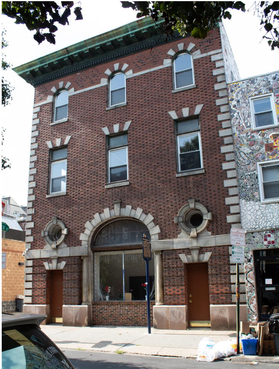
Figure 3 North elevation, 1016-18 South Street. (Source: Author, 2020)
