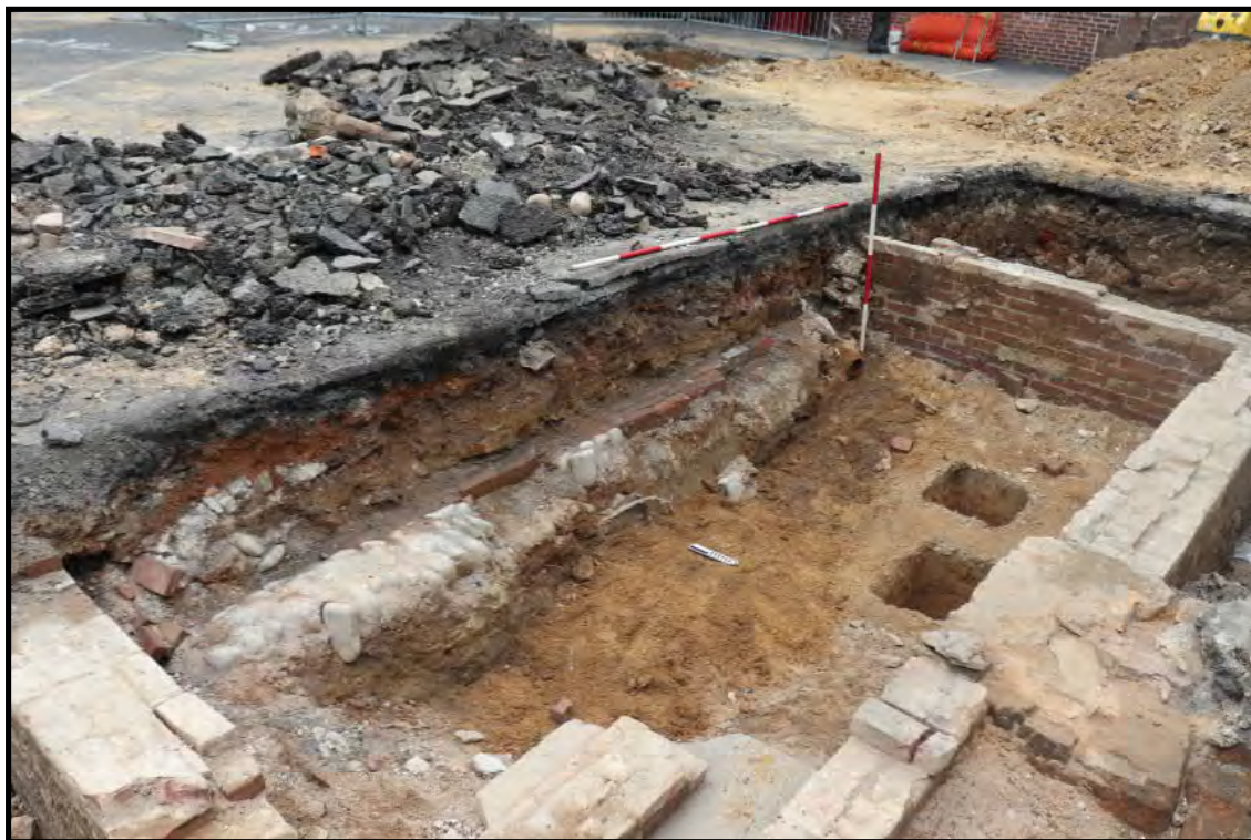
Photograph 3.15. View facing west showing the brick walls that may have formed a courtyard at the western end of the Wharton Public School in Trench 1 (Photographer: Michael Brown, July 2019) [HRI Neg.# 19027/D1:422].
