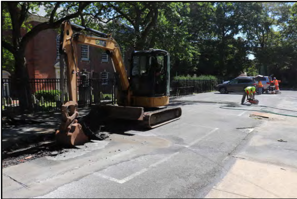
Photograph 3.1. View facing northeast showing the mechanical stripping of Test Pit A. At the mid-point of the frame the asphalt overlying Trench 1 is being cut with a road saw (Photographer: Andrew Martin, July 2019) [HRI Neg.# 19027/D1:034].
