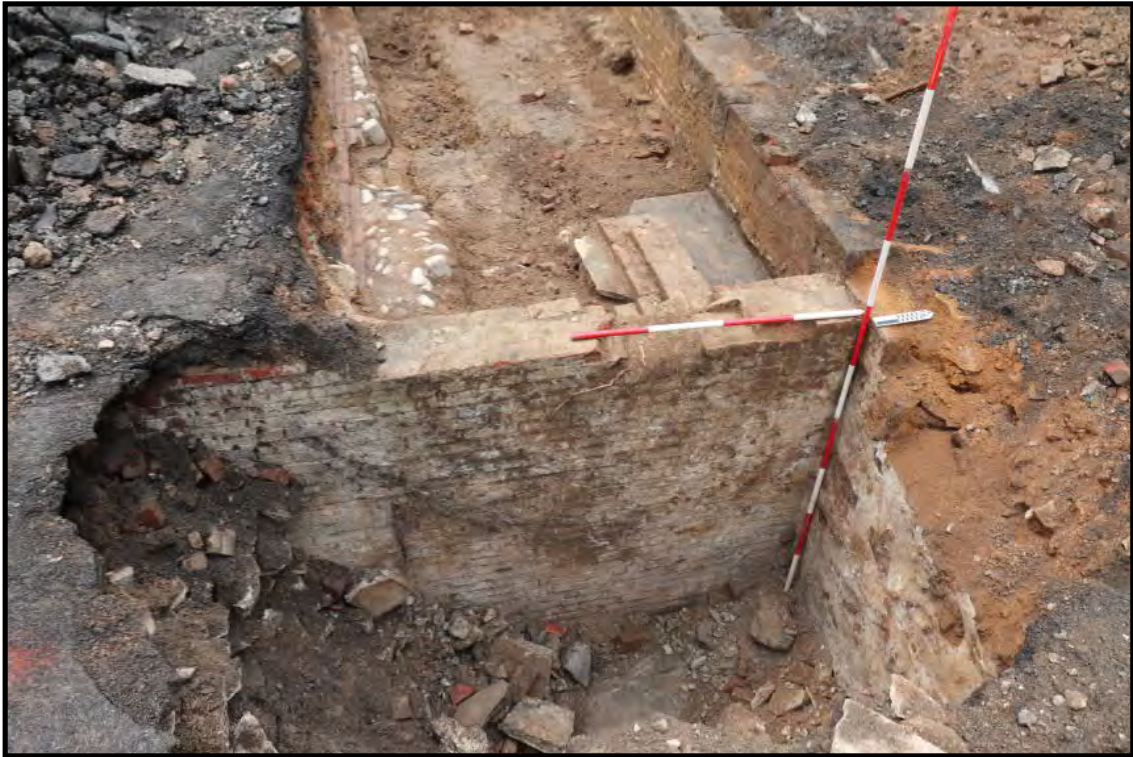
Photograph 3.13. View facing northwest showing the brick and brownstone walls of the Wharton Public School basement (Photographer: Michael Brown, July 2019) [HRI Neg.# 19027/D1:272].
