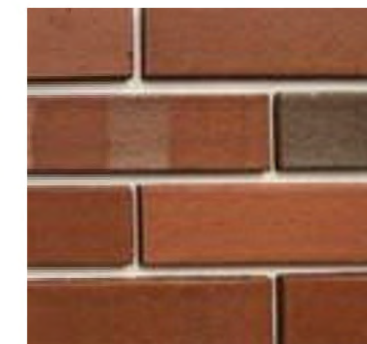
BRICK AREA 1 (LIGHTER AREA)
