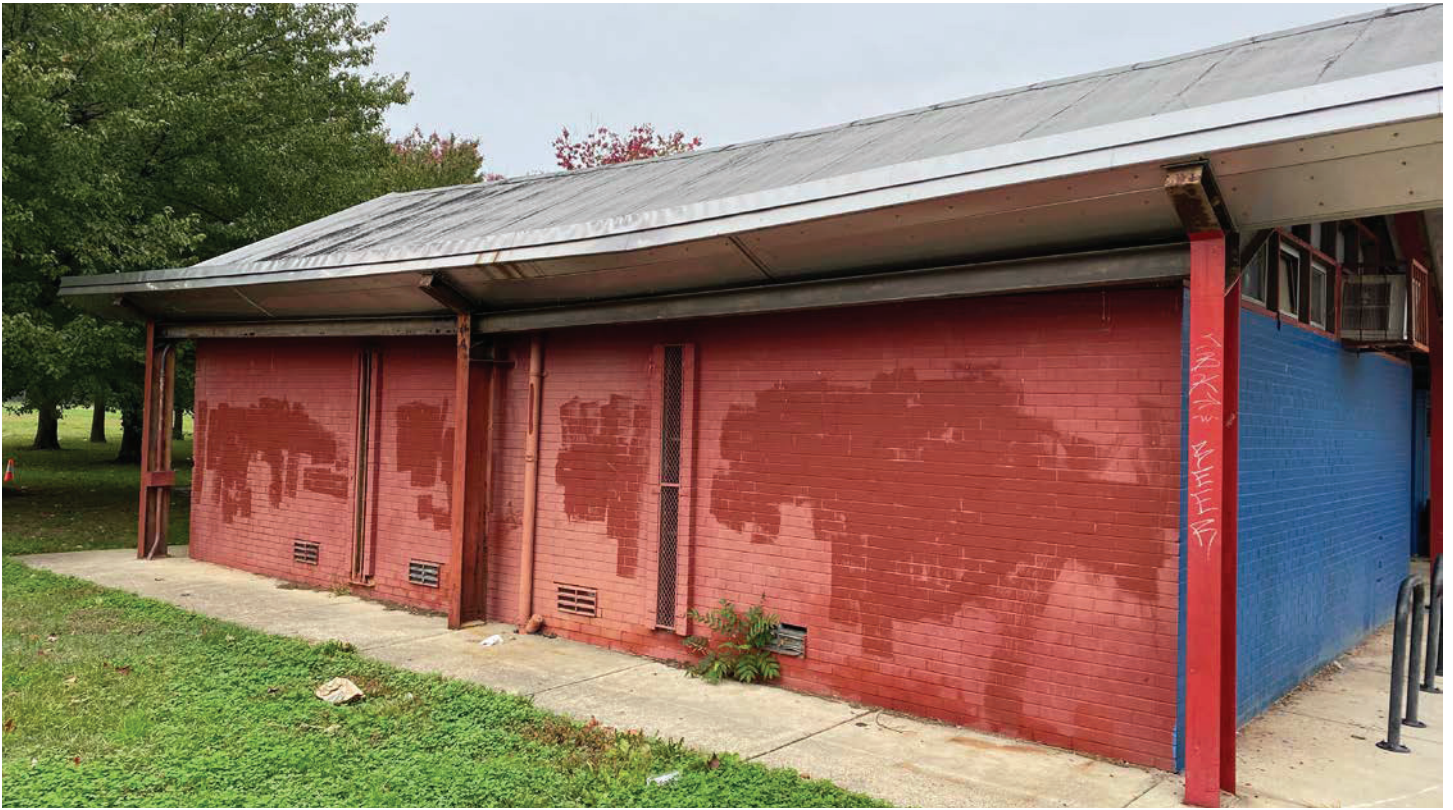
PHOTO 6: Existing south side of recreation center.
