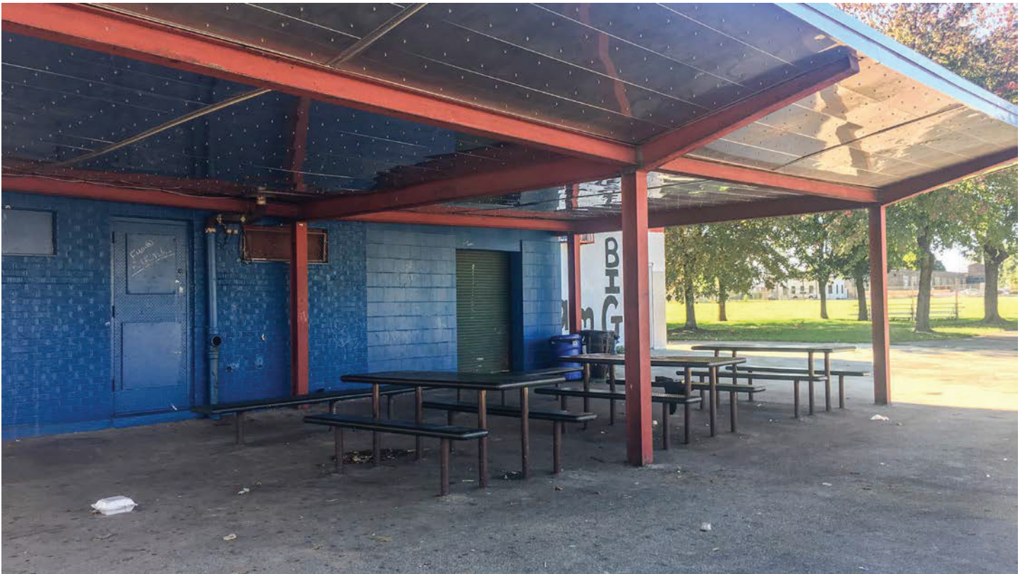
PHOTO 2: View underneath existing canopy.
