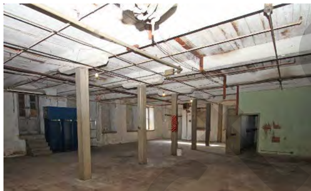
Photo 16 (left): Third floor of Mill #1 (four-story section), looking southwest. The partition at the northwest corner of this space (in green) consists of 2x4 framing with drywall, therefore it almost certainly did not exist during the tenure of Benjamin W. Greer.
