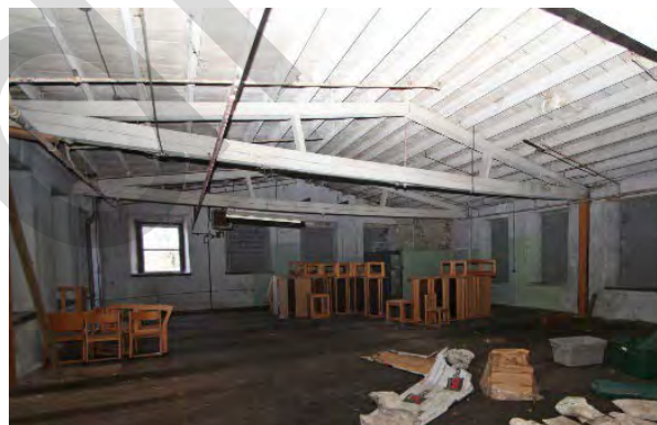
Photo 16 (left): Third floor of Mill #1 (four-story section), looking southwest. The partition at the northwest corner of this space (in green) consists of 2x4 framing with drywall, therefore it almost certainly did not exist during the tenure of Benjamin W. Greer.
