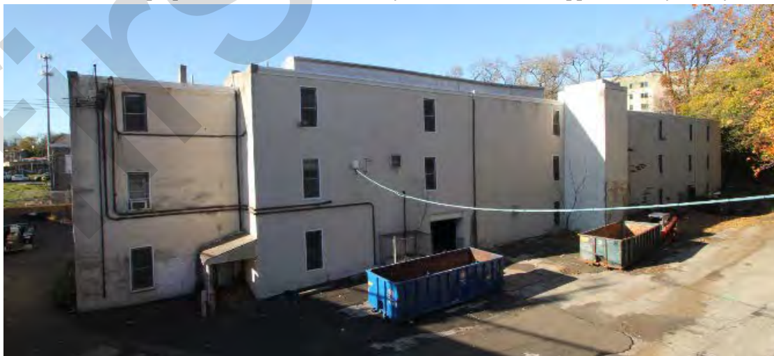
Photo 1: East elevation of Mill #1, looking northwest from Belfield Avenue. The rooftop monitor on the southern half of Mill #1 is visible in this view. The square tower on the east elevation contains an elevator shaft.
