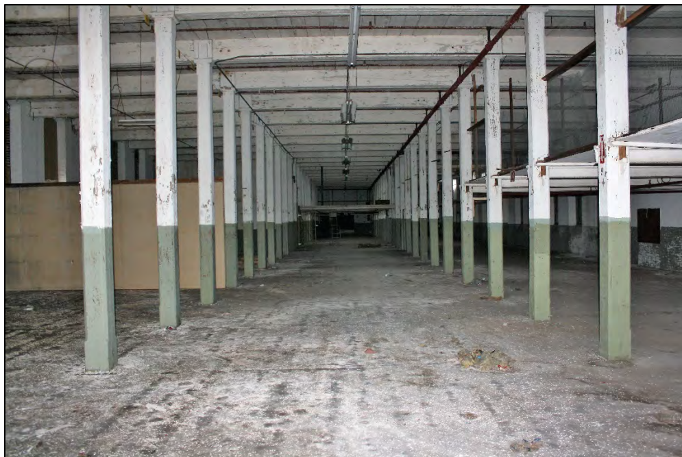
PHOTOGRAPH 26 – Building 2 – third floor interior looking north between the two rows of wood, square columns.
