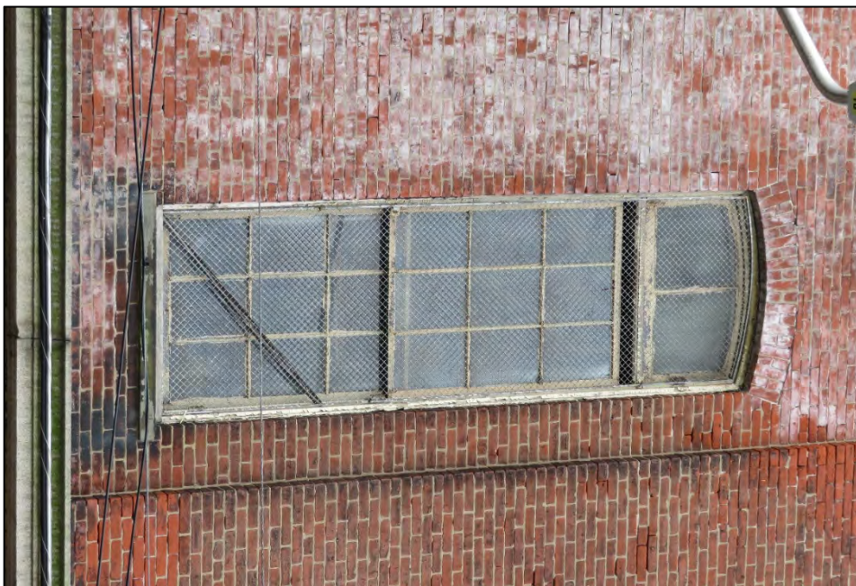
PHOTOGRAPH 5 – Annex, north (front) elevation, second floor, Bay 13, with typical nine-over-nine, double hung wood sash with a two-light, segmental arched transom.
