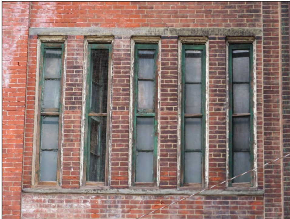
PHOTOGRAPH 10 – Building 1, south (rear) elevation, second floor wood casement windows that are set between stone lintels and sills.
