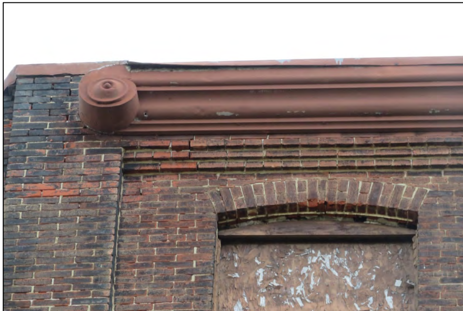
PHOTOGRAPH 11 – Building 1, south (rear) elevation, parapet with a painted, galvanized metal cornice at the head of the corbelled blind panel
