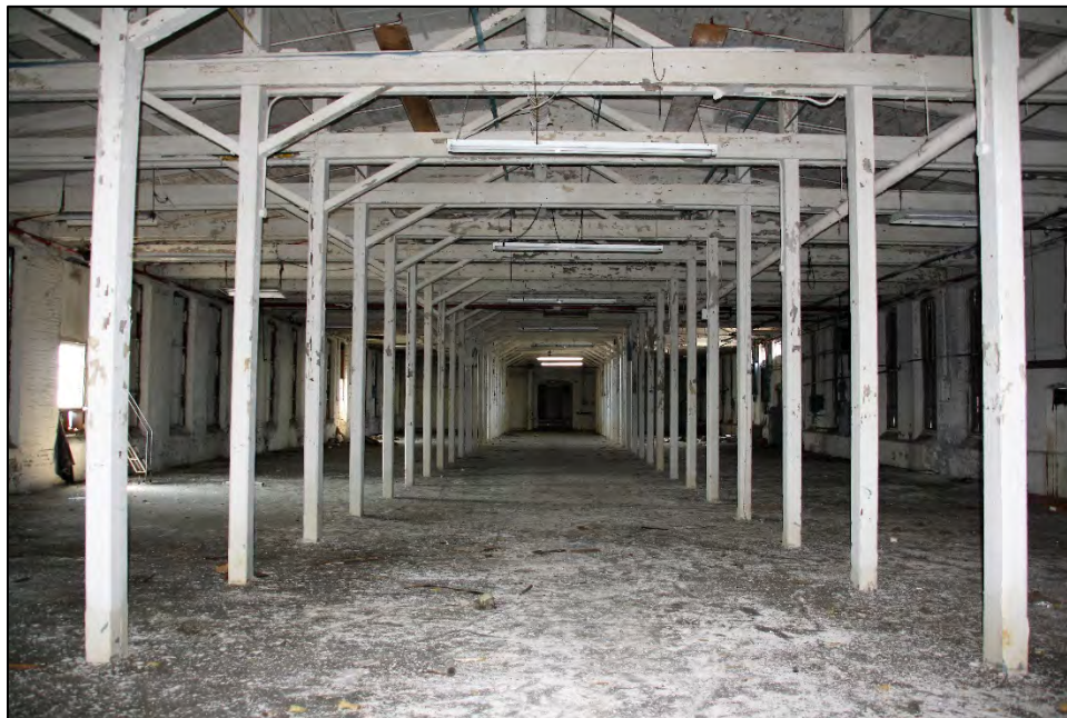
PHOTOGRAPH 31 – Building 2 – fifth floor interior looking south with the roof deck trusses that extend below the beams.
