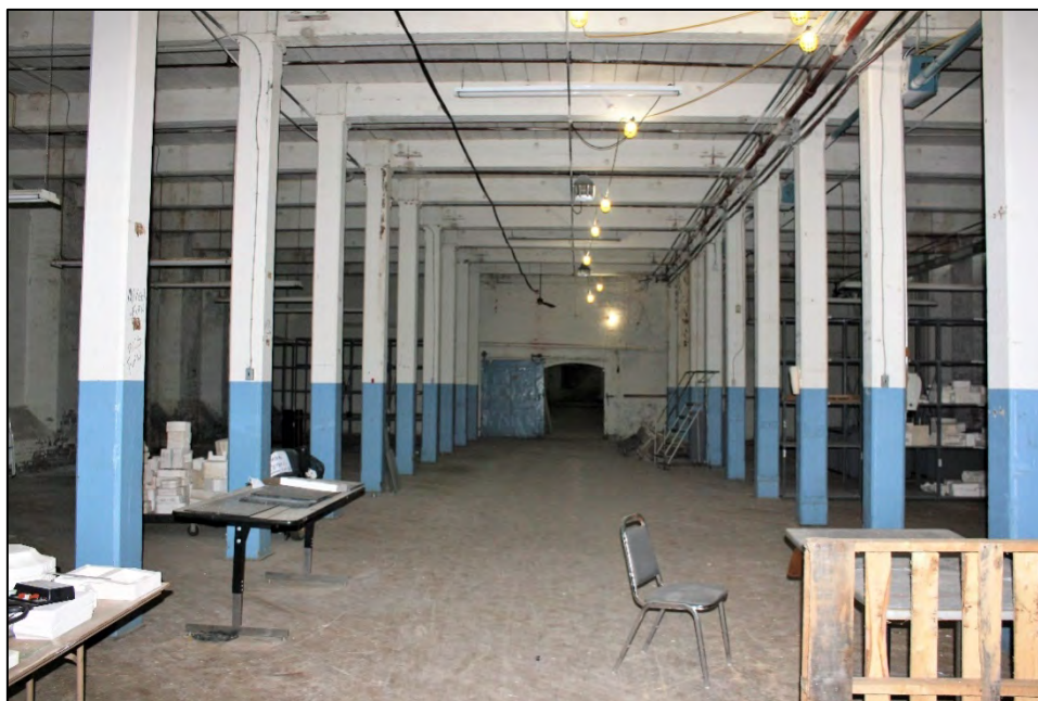
PHOTOGRAPH 21 – Building 2 – first floor interior looking south between the two rows of square, wood columns.
