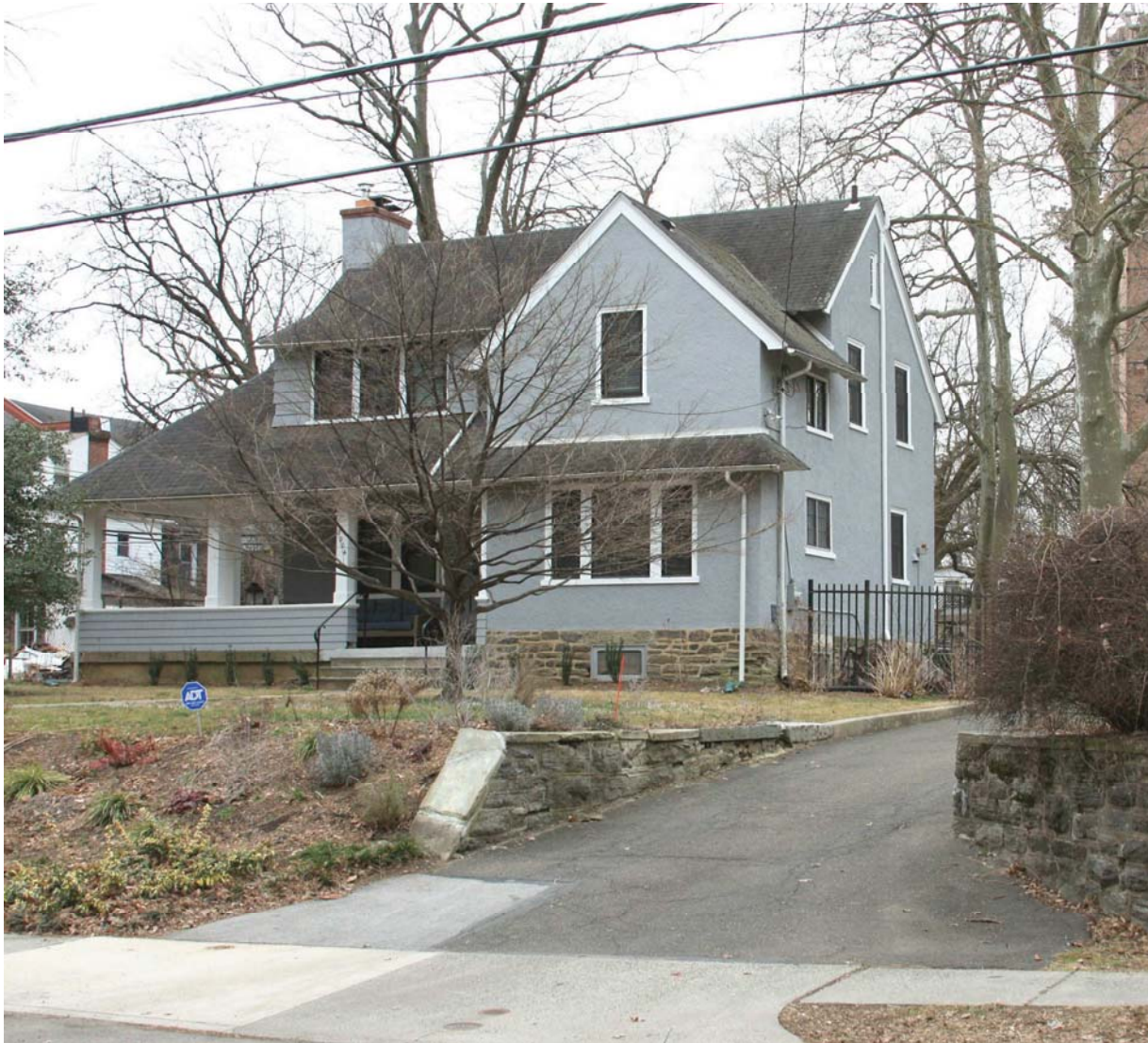
NORTH AND WEST FACADE FROM BOYER STREET
