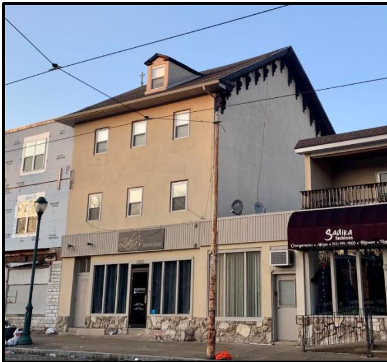
Figure 4. Top: Looking northeast at the subject property's primary (southwest) elevation. Figure 5. Bottom: Looking north at the subject property's primary (southwest) and side (southeast) elevations. Courtesy Oscar Beisert.
