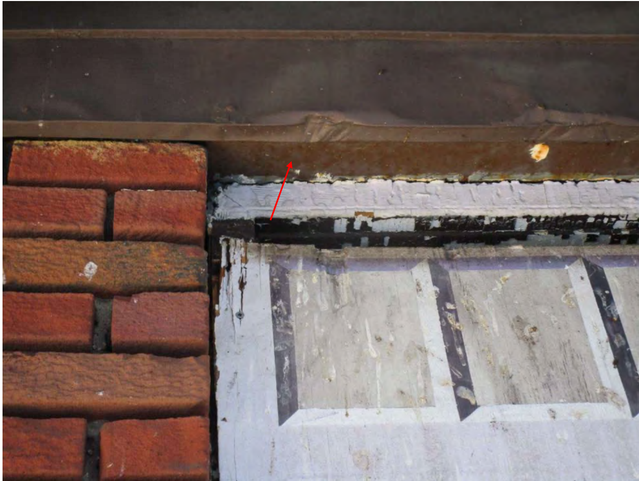
Photo 44: Failed coating and surface corrosion at steel lintel
