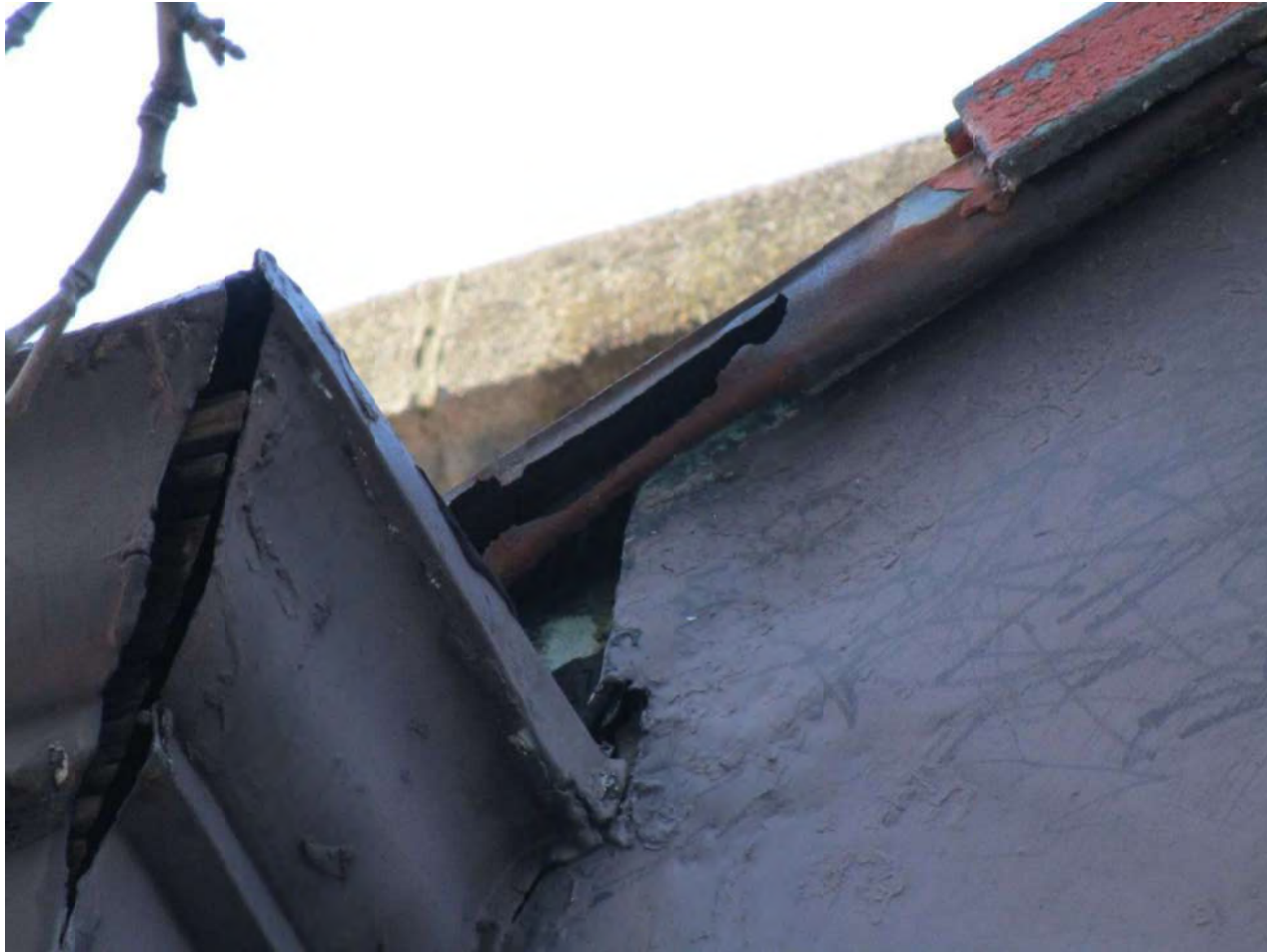
Photo 26: Section loss in metal roof element
