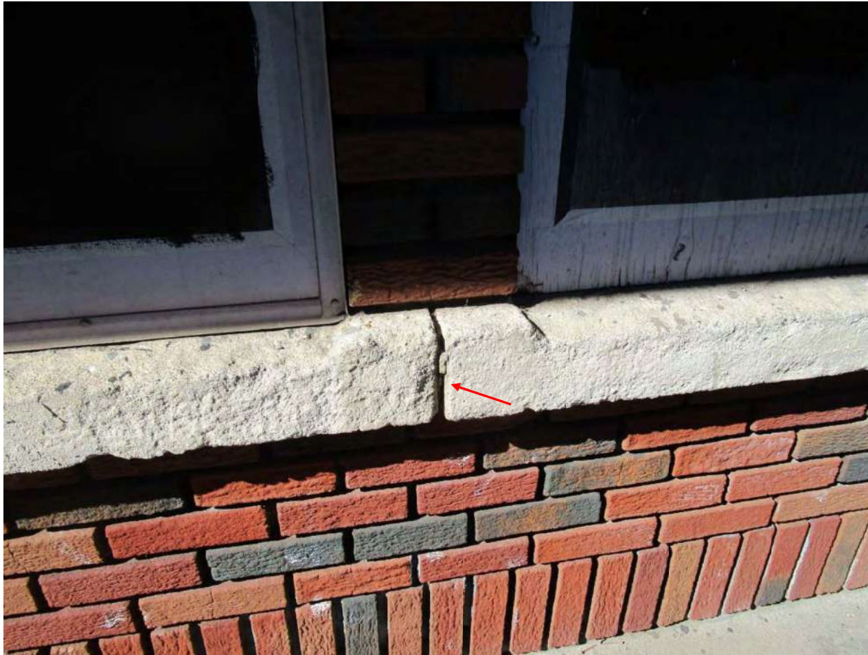
Photo 39: Deteriorated mortar joint in cast stone sill
