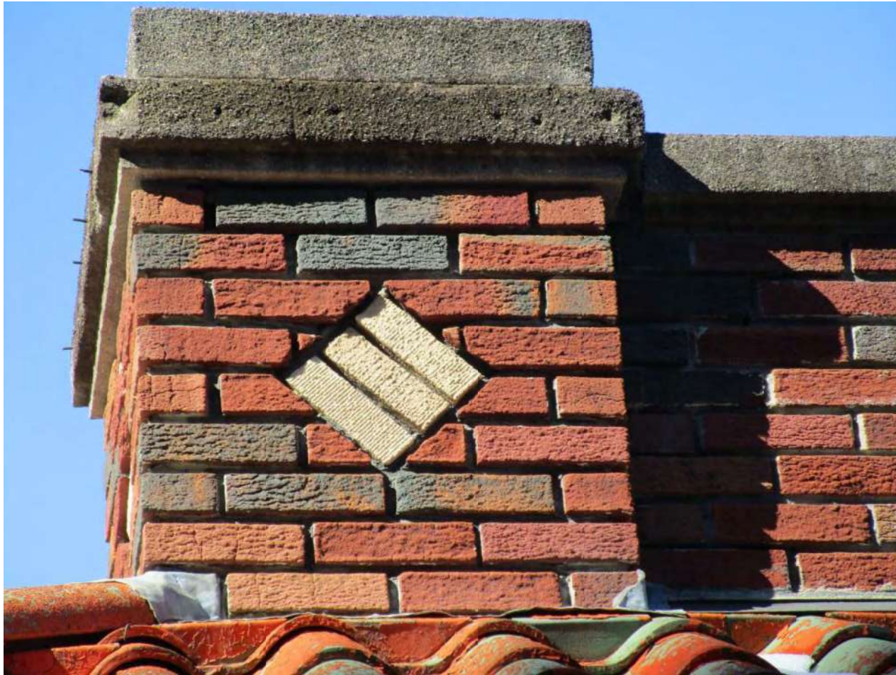
Photo 33: Surface erosion at brick face & deteriorated mortar joints
