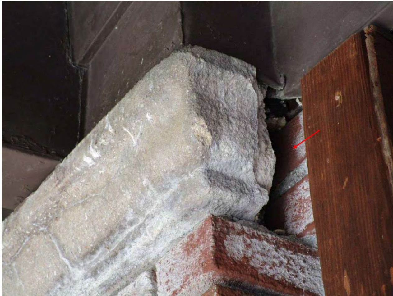
Photo 36: Spall and section loss in cast stone capital
