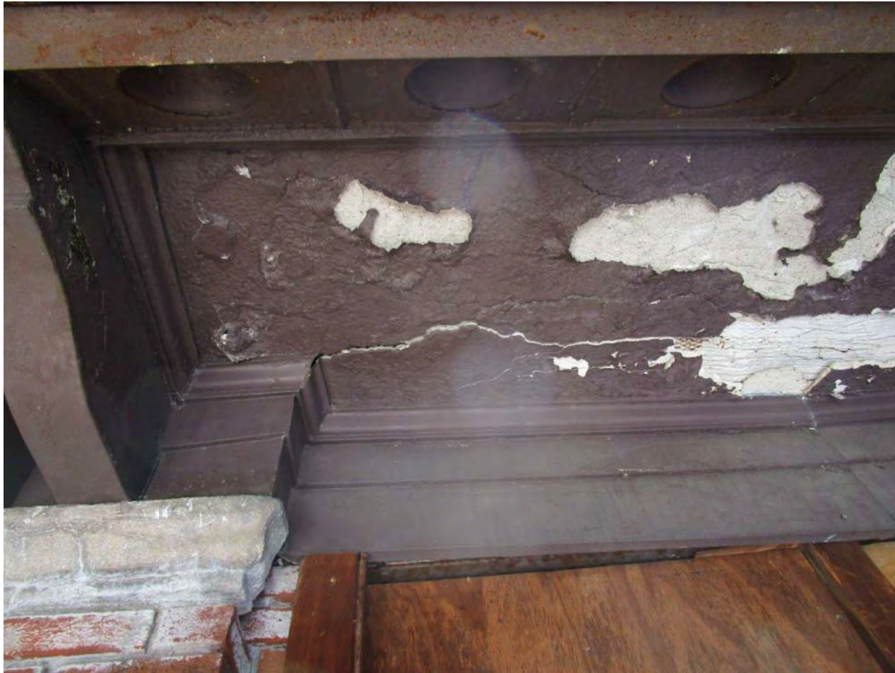
Photo 29: Failed plaster
