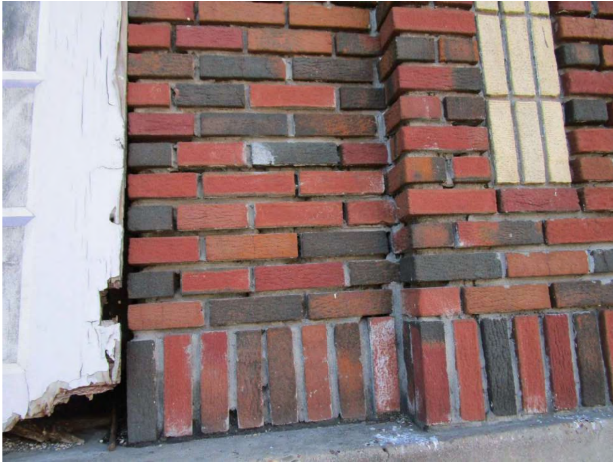
Photo 35: Surface erosion at brick face & deteriorated mortar joints
