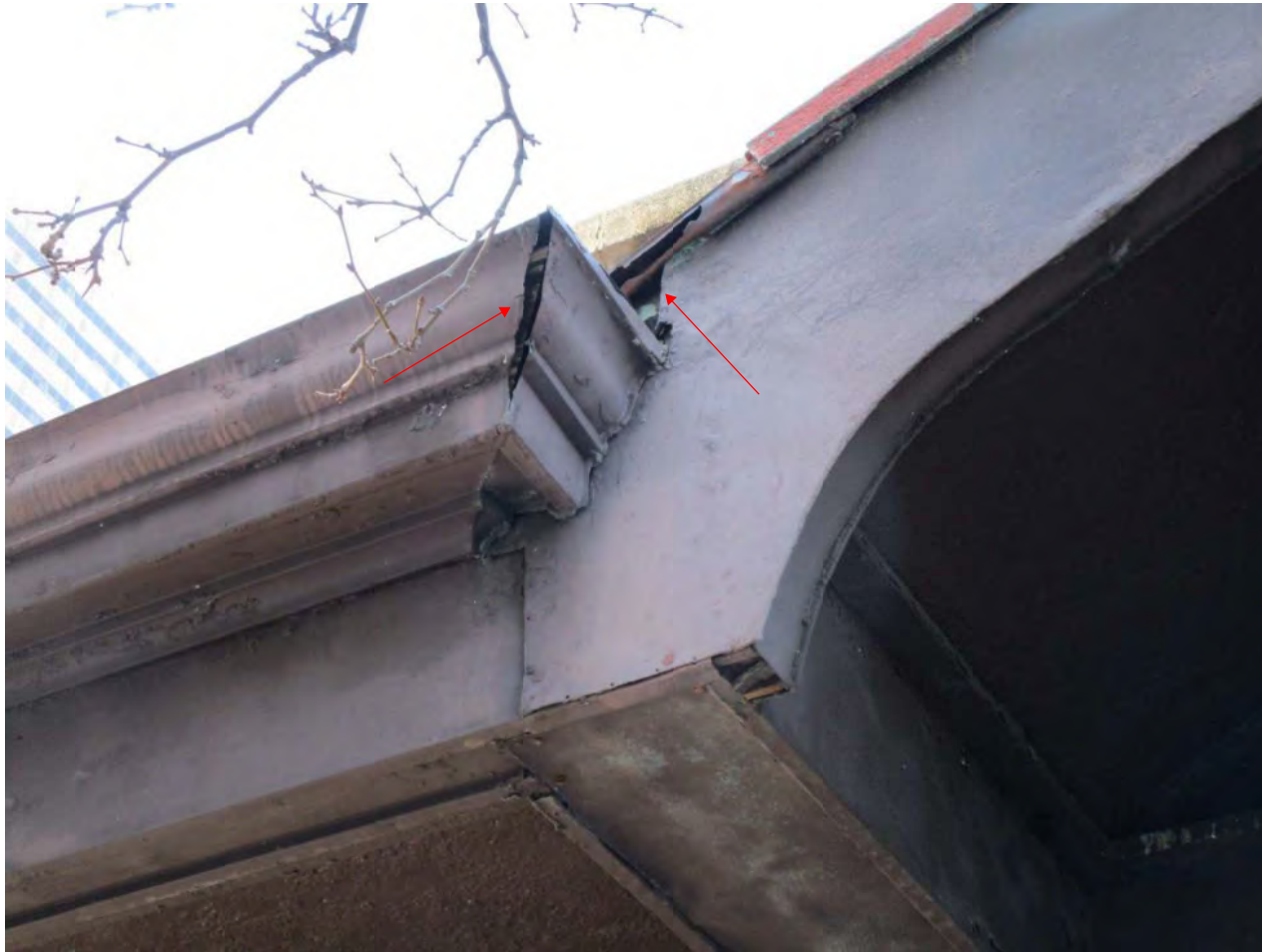
Photo 25: Opening in pent eave cornice
