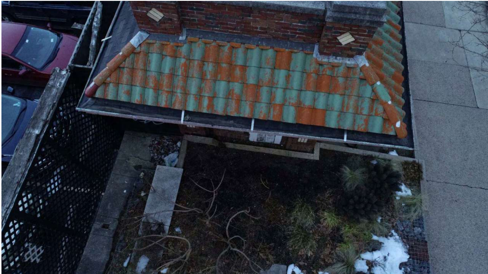
Photo 46: Failed orange paint at green terra cotta tiles
