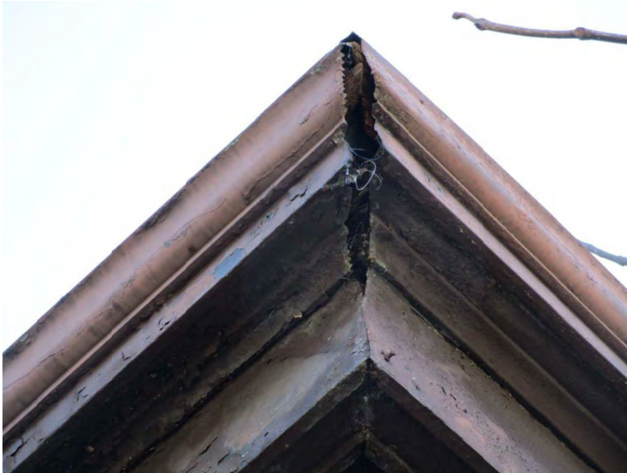
Photo 27: Opening in pent eave cornice
