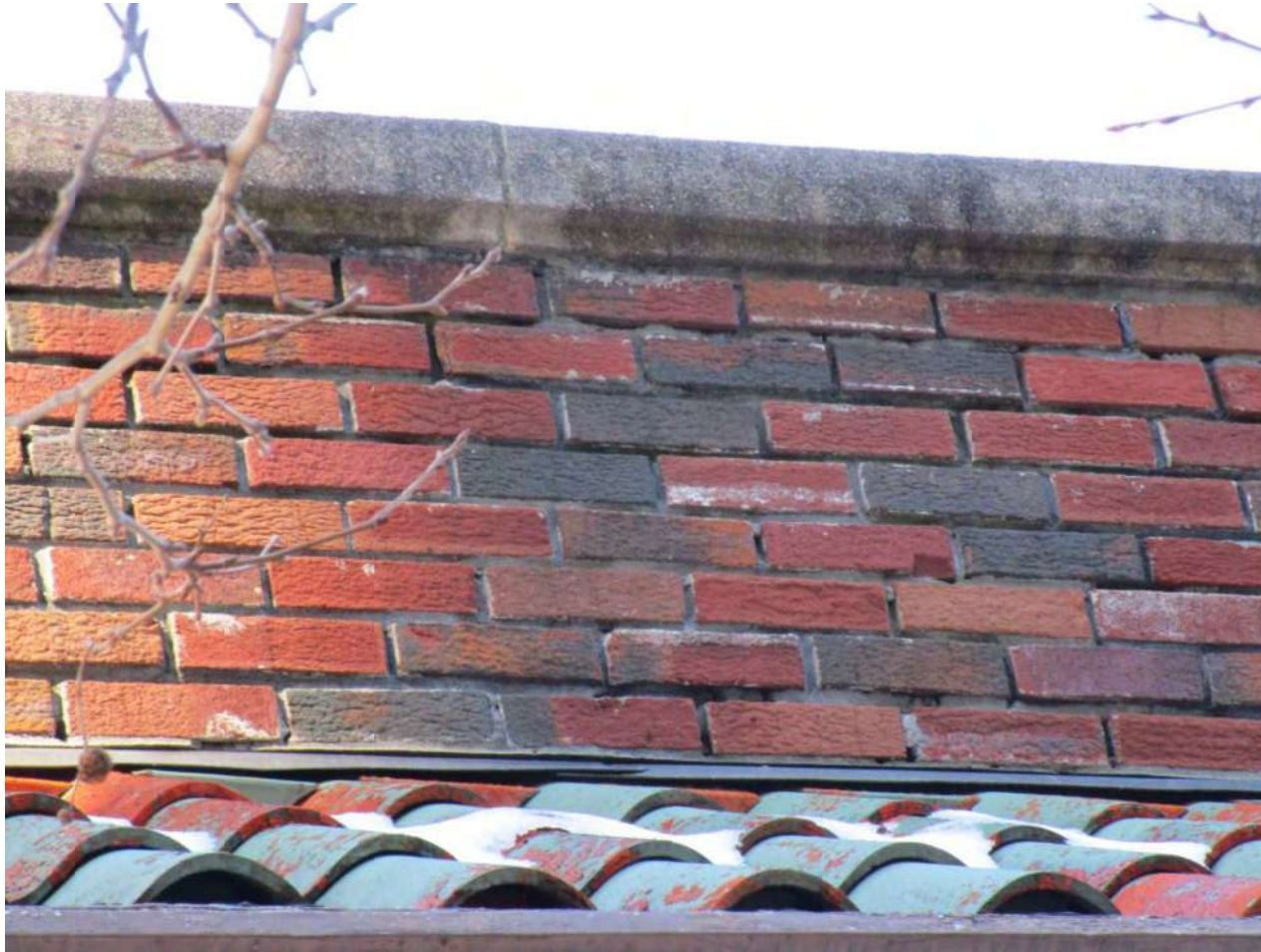
Photo 34: Surface erosion at brick face & deteriorated mortar joints
