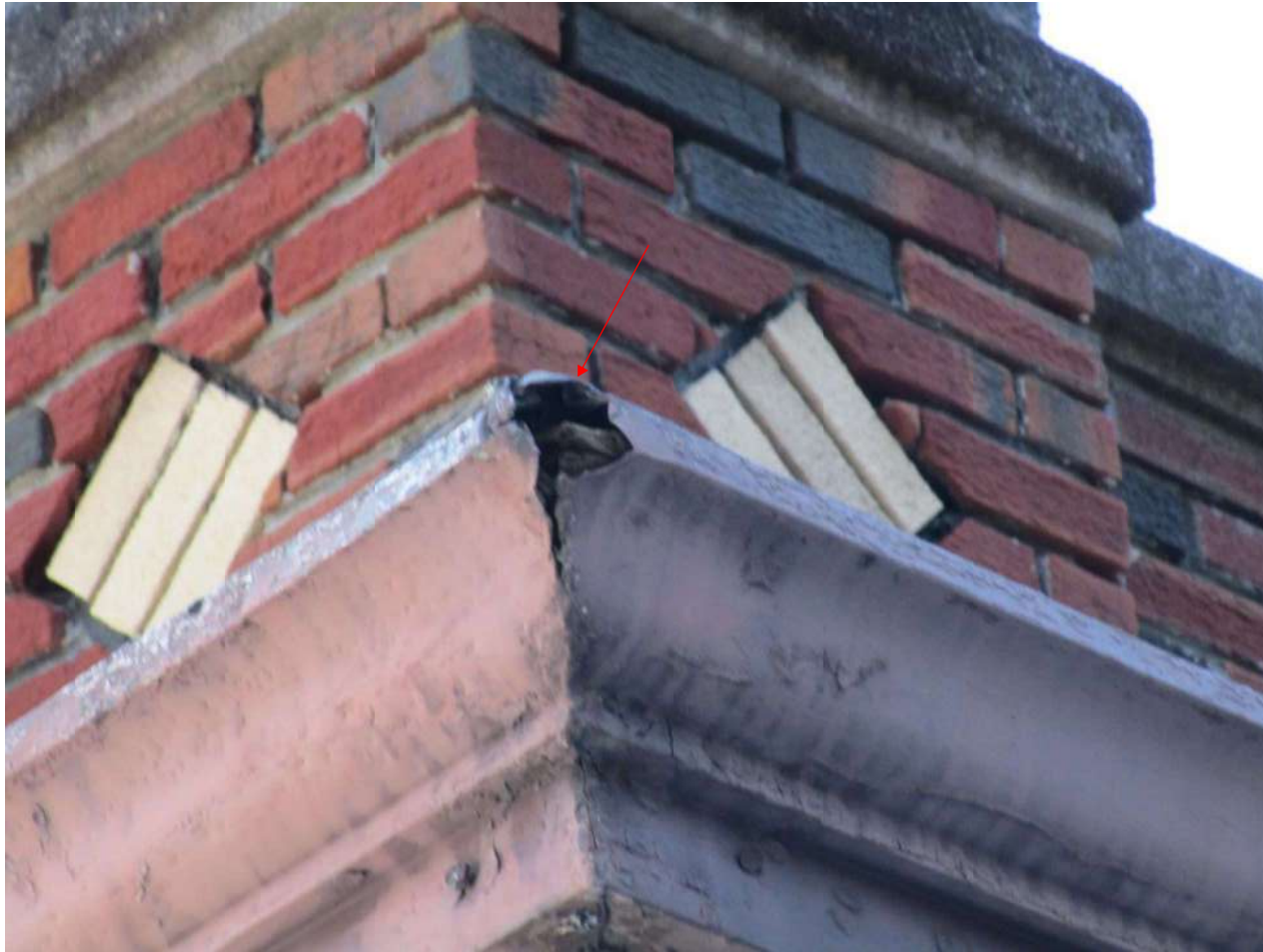
Photo 24: Section loss of pent eave cornice. Failed wood framing.
