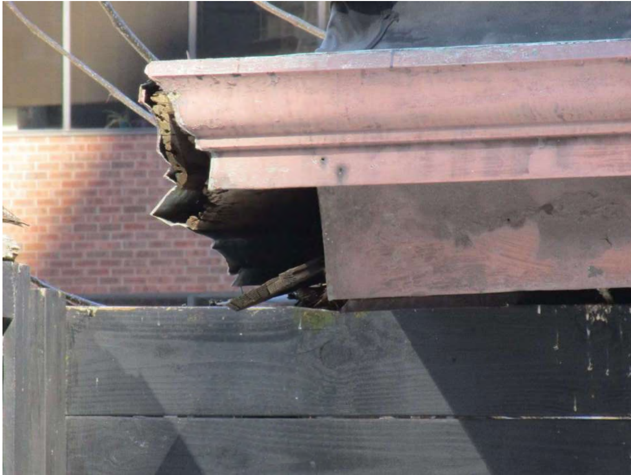
Photo 23: Section loss and displacement of pent eave cornice. Failed wood framing.
