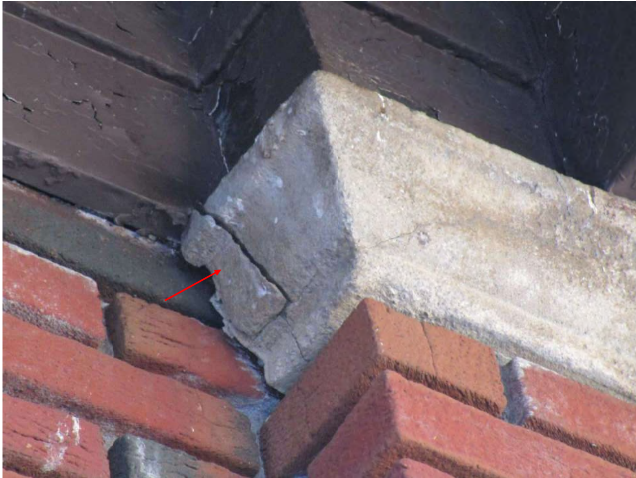
Photo 37: Spall in cast stone capital
