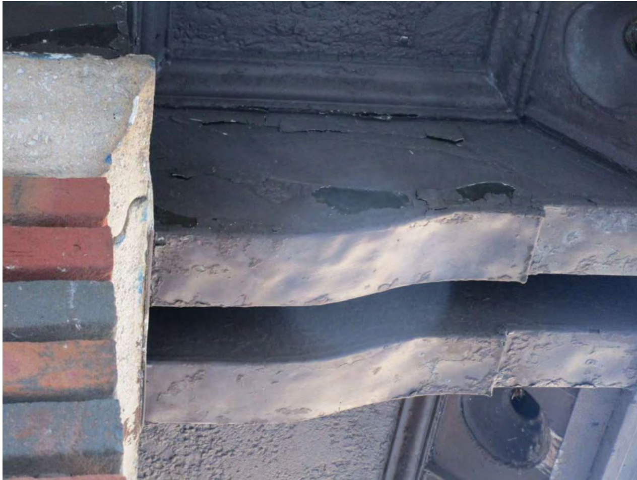
Photo 32: Failed coating and surface corrosion
