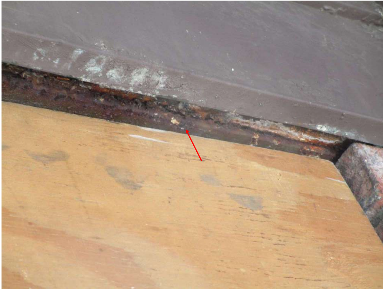
Photo 42: Failed coating and surface corrosion at steel lintel
