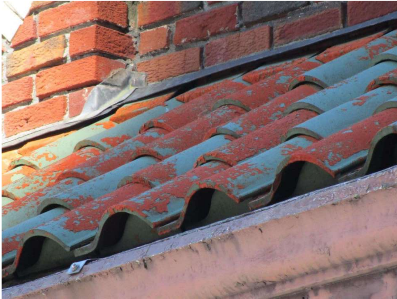
Photo 45: Failed orange paint at green terra cotta tiles
