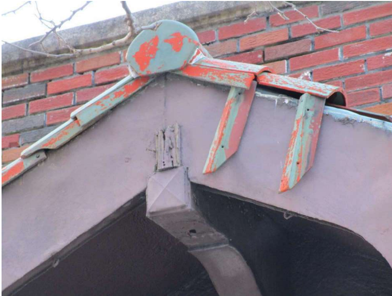
Photo 48: Loose and displaced terra cotta tiles
