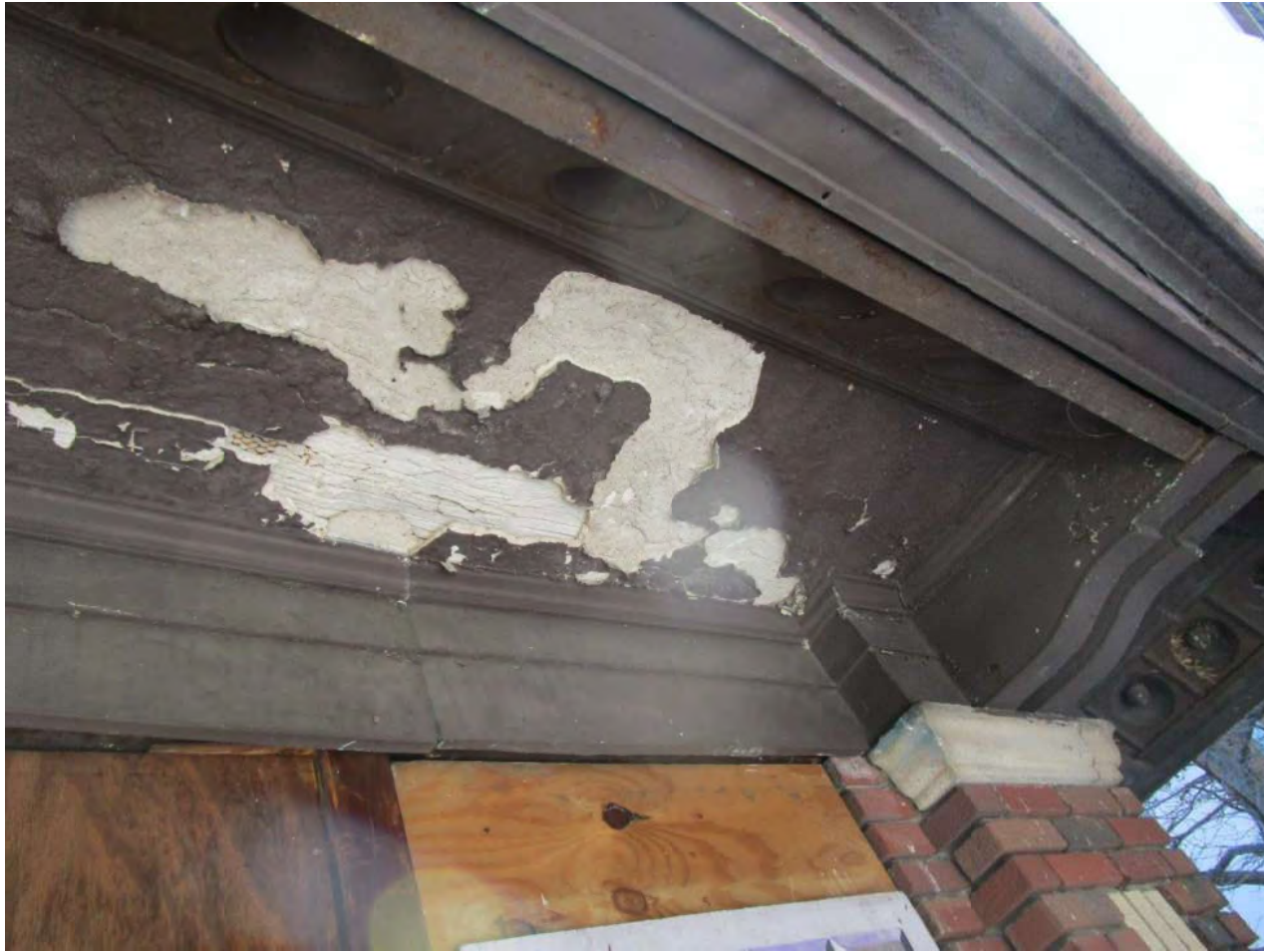
Photo 30: Failed plaster
