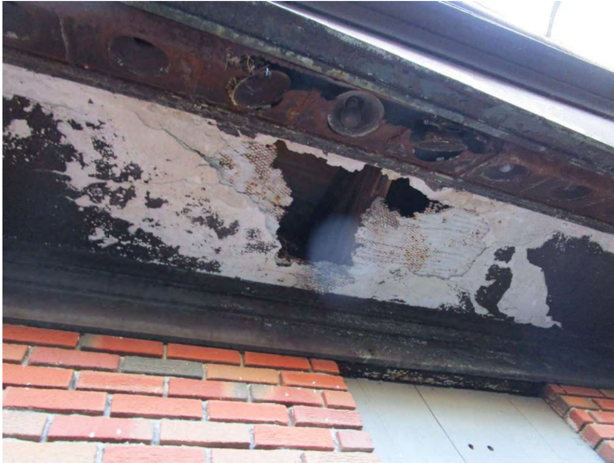
Photo 31: Failed plaster and section loss at light fixture
