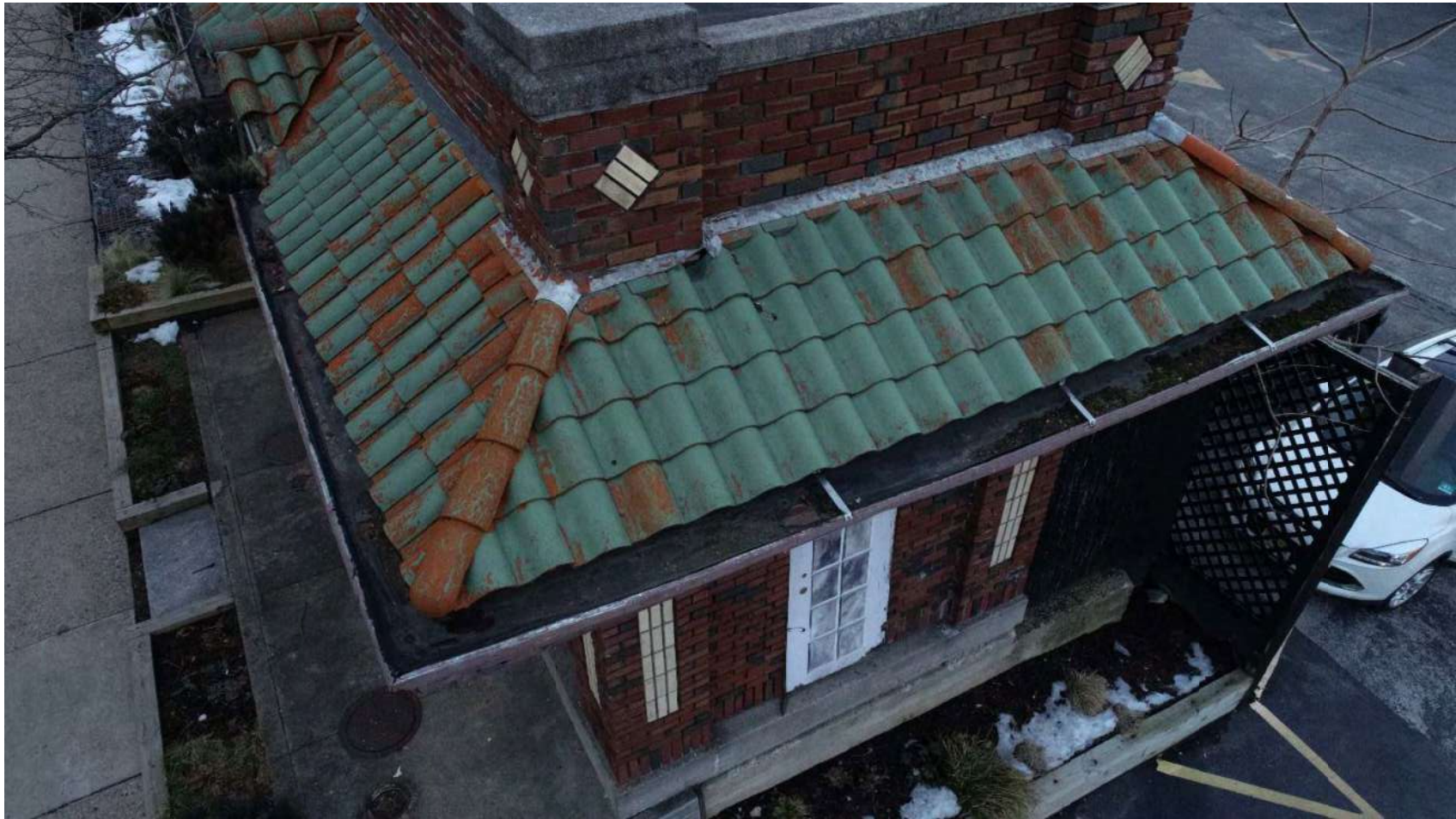
Photo 47: Failed orange paint at green terra cotta tiles
