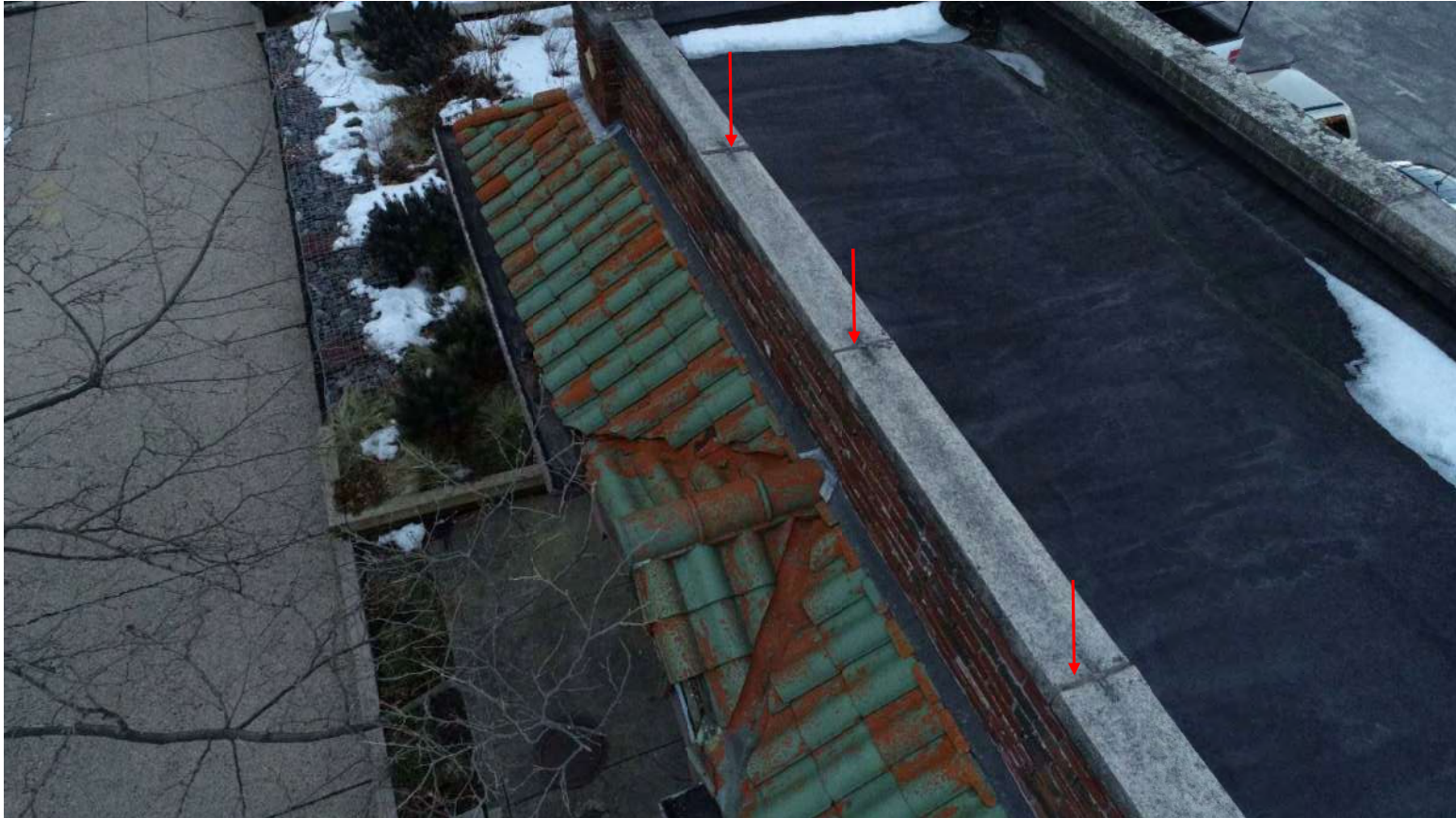
Photo 41: Deteriorated sky-facing joints in coping stones
