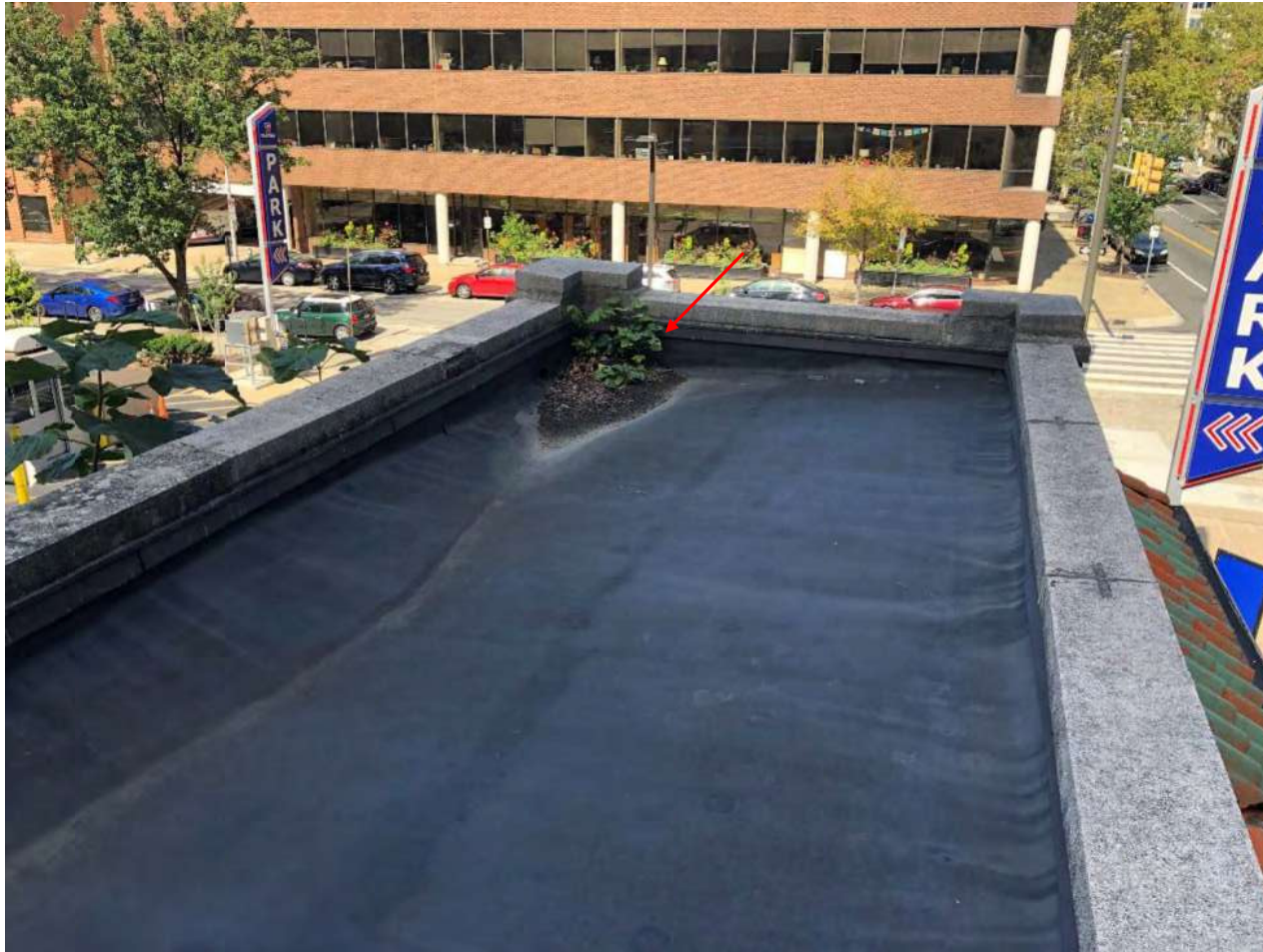
Photo 49: Biological growth at EPDM flat roof
