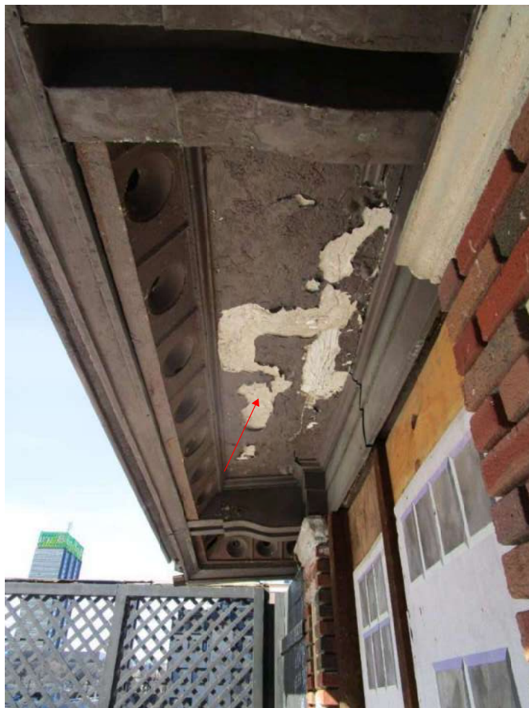
Photo 28: Failed plaster
