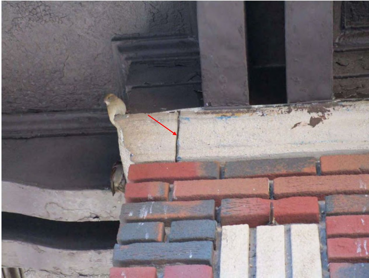
Photo 40: Deteriorated mortar joint in cast stone capital
