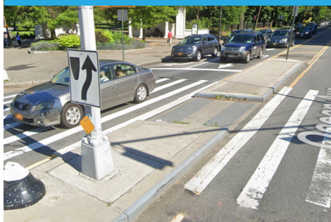
Cut-through Concrete Median
