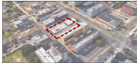
3 LOOKING SOUTH-WESTWARD TOWARDS SITE
