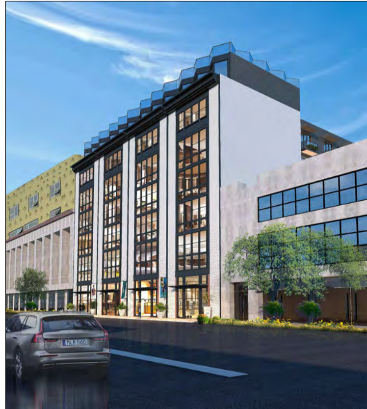
LOOKING NORTHWARD ON N BROAD ST
