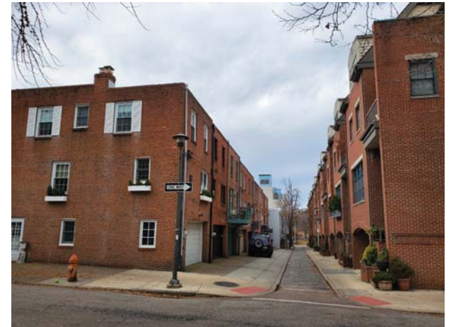
5 View from sidewalk looking west at the 2500 block of Panama Street
