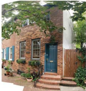
Existing Front Facade - View from sidewalk looking east. (ca September 2020) Note: Photographic distortion due to panorama; existing buildings are not curved.
