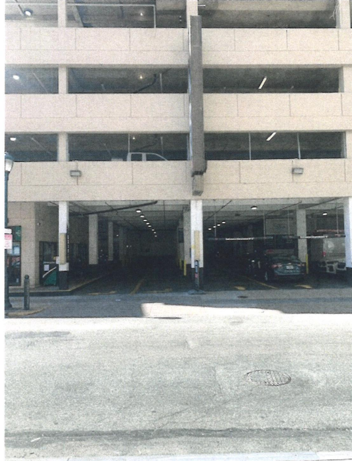
Looking across the street
