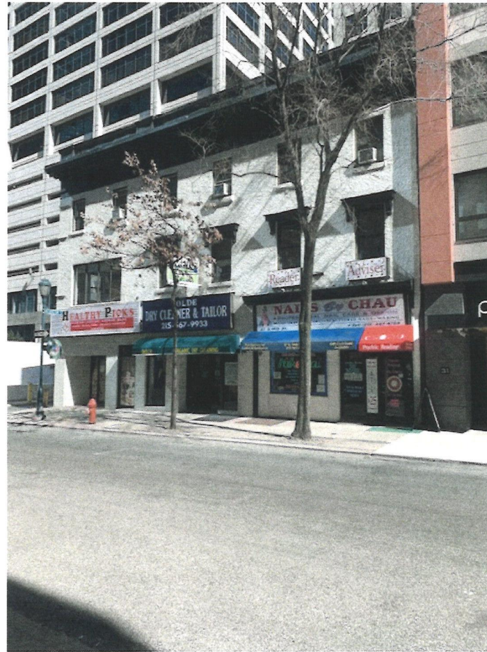
Front elevation – building to left
