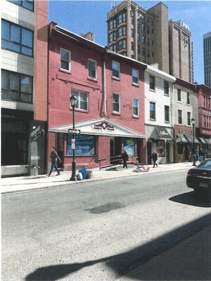
Front elevation – building to right
