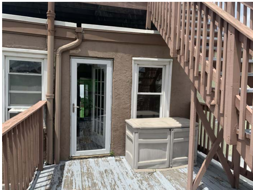
EXISTING DECK: INTERMEDIATE LEVEL, LOOKING TOWARD ACCESS DOOR AT REAR
