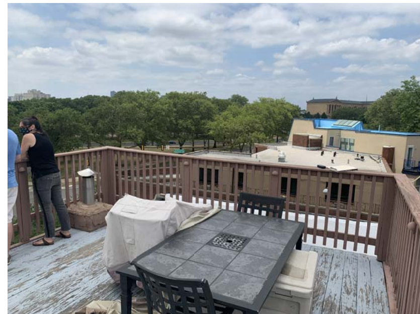
EXISTING DECK: UPPER LEVEL, LOOKING SOUTH
