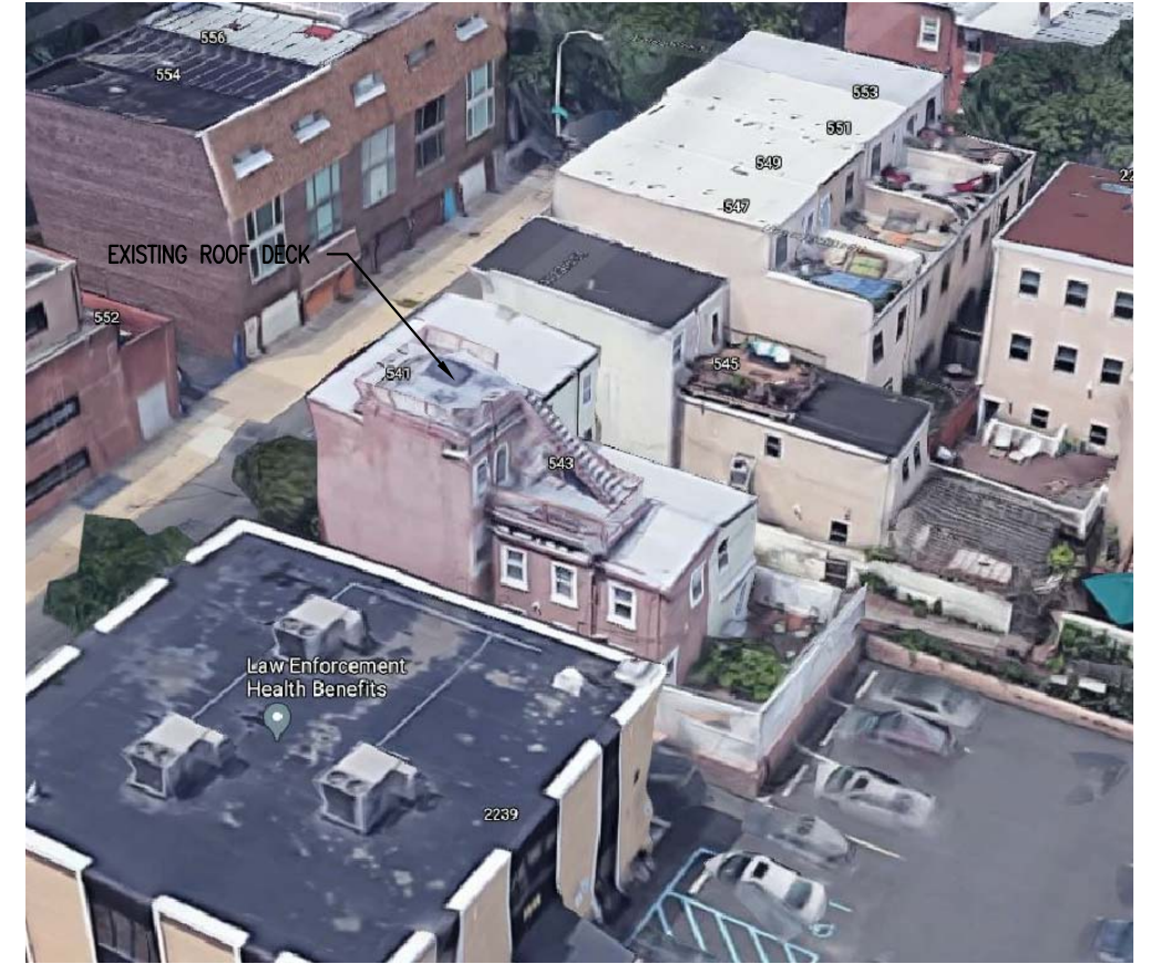
AERIAL VIEW: LOOKING NORTHWEST
