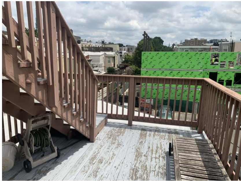
EXISTING DECK: INTERMEDIATE LEVEL, LOOKING EAST
