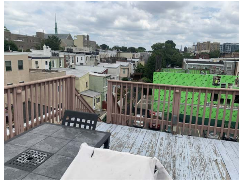
EXISTING DECK: UPPER LEVEL, LOOKING EAST
