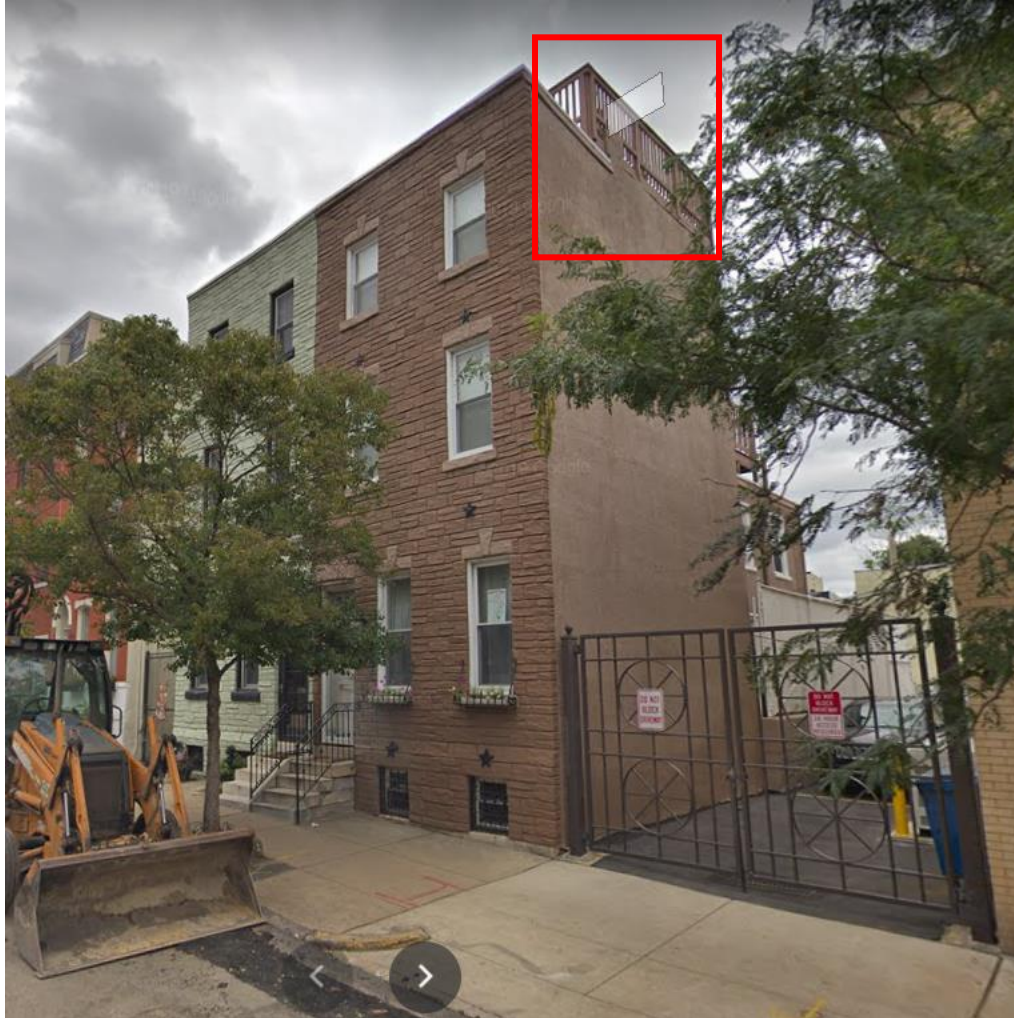
Image 1. View of roof deck from street. Google Streetview.
