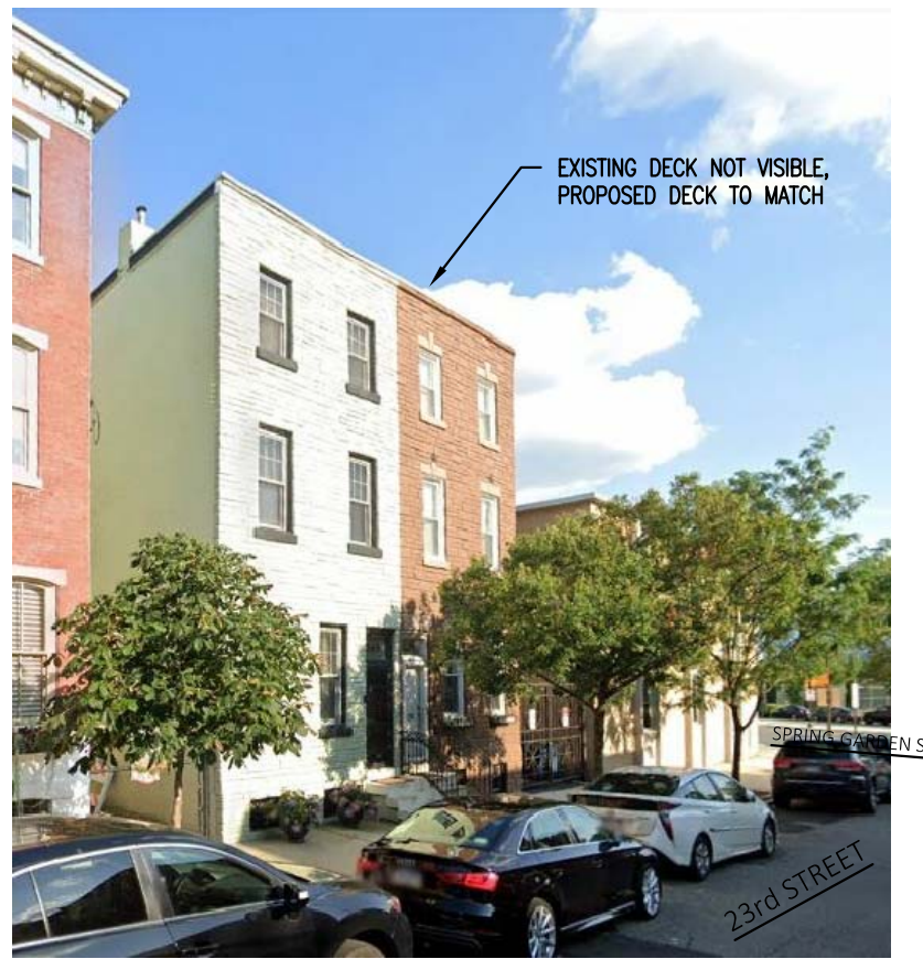
STREET VIEW: LOOKING SOUTHEAST
