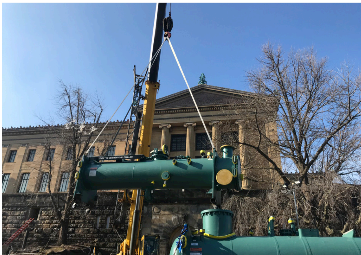
Workers outside the Philadelphia Museum of Art lift a new high efficiency chiller off the delivery truck.
