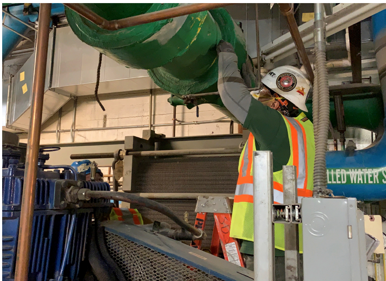
Workers installing a new energy efficient chiller at the Philadelphia Museum of Art.
