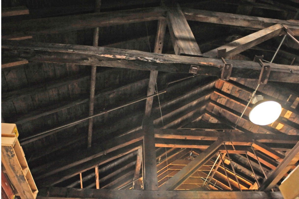
Building 2: Black rot, white fungi, and charring on roof planking, reconstruction at far end (right)
