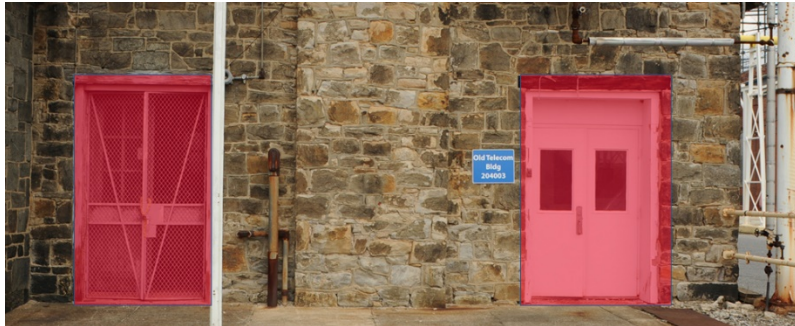
Altered windows and door openings: Gothic door and paired Gothic windows turned into modern doors, Building 1a.
