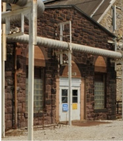
Much altered façade Building 5b, frames, windows removed
