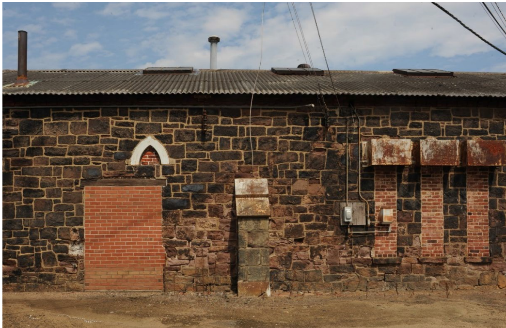
Shop building alterations: windows infilled and enlarged into doors, later infilled with brick; extensive masonry damage from erosion
