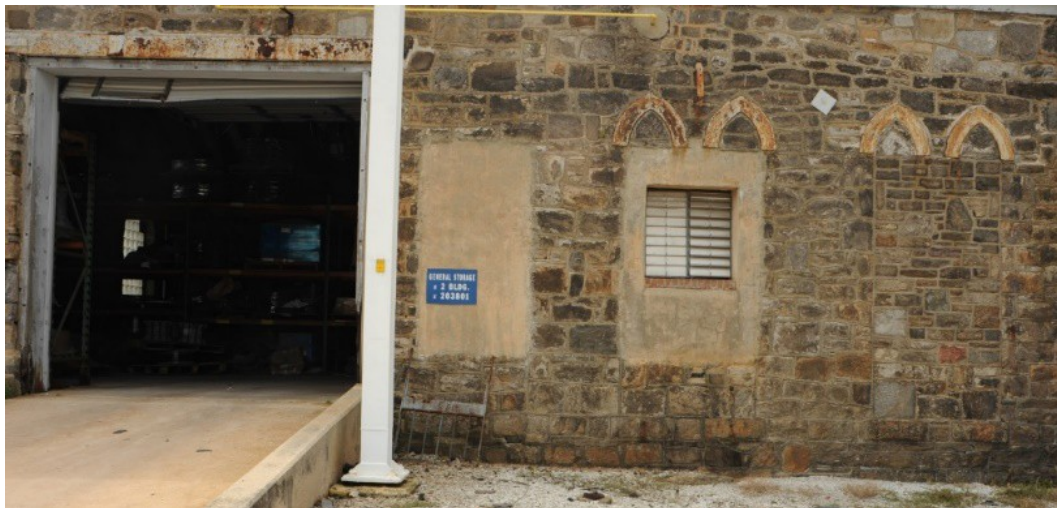
Building 1 b, rear wall, every opening altered because of inadequacy for later uses, resulting in loss of integrity
