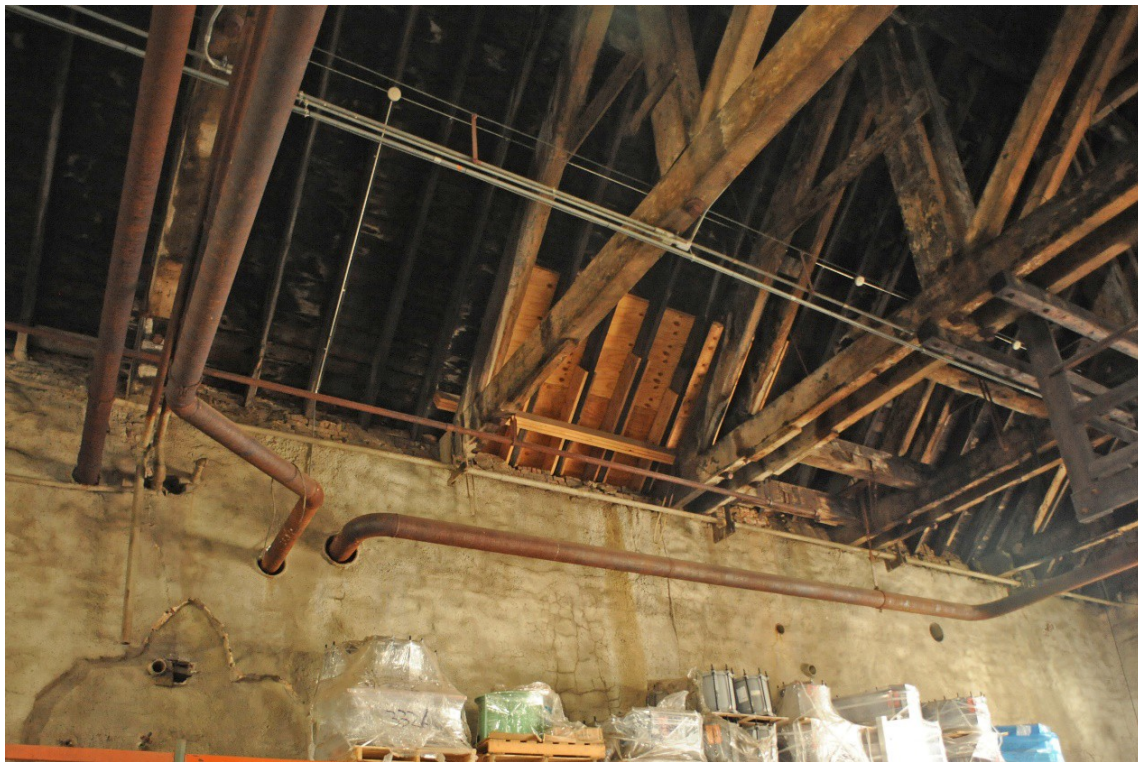
Building 5 roof damage—black are as show rot and charring from fires, replacement trusses and plywood sheathing
