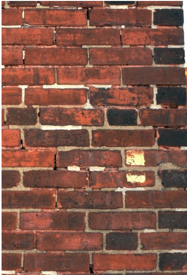
Garage wall, common brick with failing brick surface
