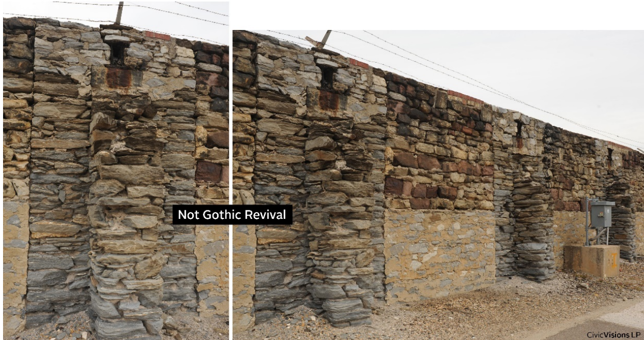
The buttresses of the wall fragment of the long-since demolished coal storage building are simply present to stabilize masses of coal under shelter.
