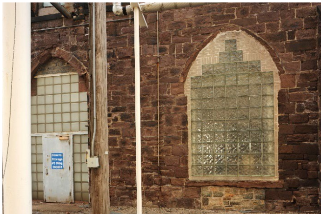
Door and window frames removed; masonry hoods shaved off, glass block infill. Left: Building 5a; Right: Building 2
