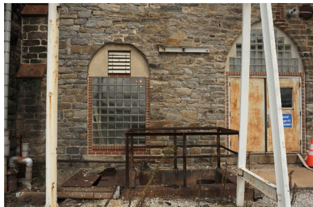
Door and window frames removed; masonry hoods shaved off, glass block infill. Left: Building 5a; Right: Building 2
