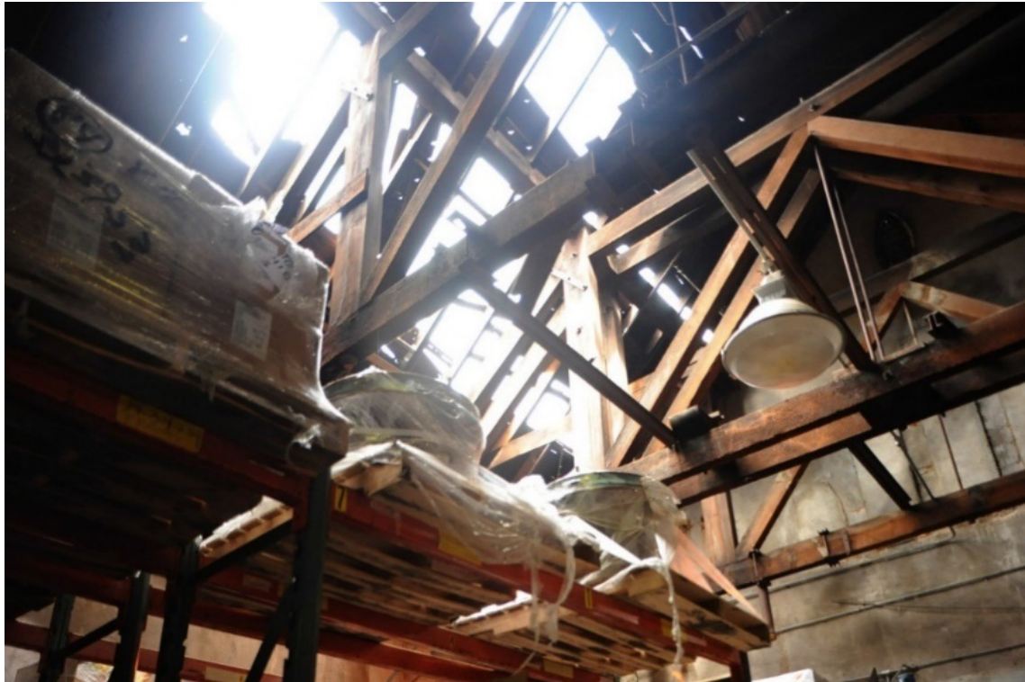
Building 5, roof damage in windstorm, summer 2020 with roof sheathing blown out
