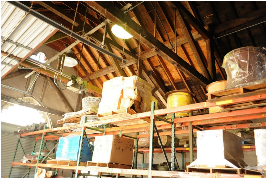
Building 2 previous roof repairs and reconstruction, replacement truss and plywood roof underlayment on left (Building 2)
