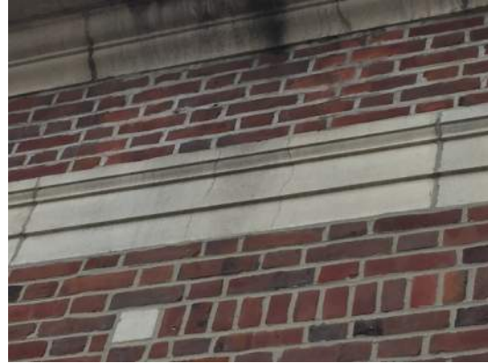
Photograph #12: Stress cracks in entablature
