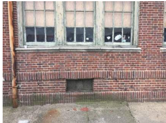
Photograph #6: Typical rust jacking at ground level windows with excessive cracking
