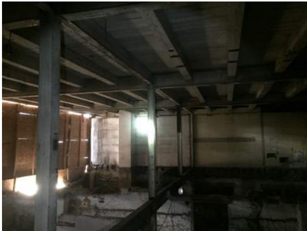
Photograph #21: Second Floor Framing
