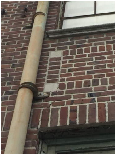
Photograph #5: Front brick cracks at jamb NE corner
