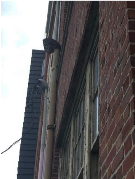
Photograph #7: Bowing of brick
