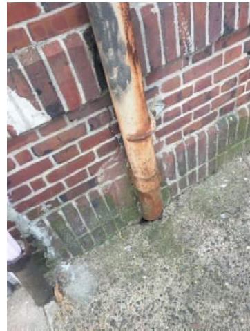
Photograph #4: NE Corner brick cracks at broken storm pipe
