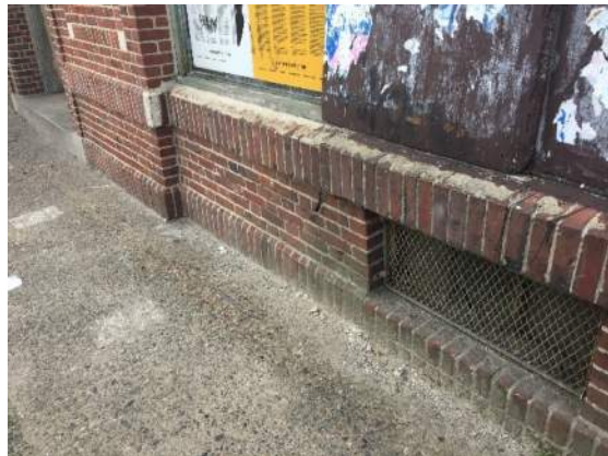
Photograph #10: Additional rust jacking at ground level window
