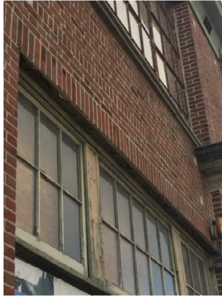
Photograph #8: Bowing of brick and leaning of wall
