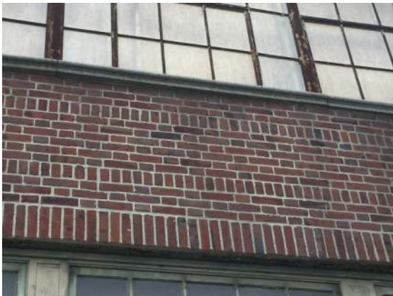
Photograph #9: Cracking and distress at 2 nd floor sill
