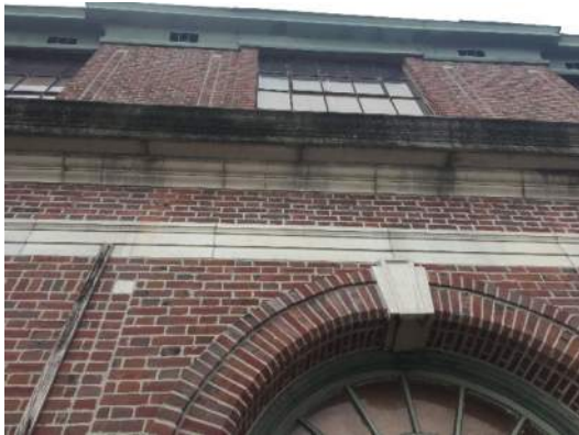
Photograph #13: Water infiltration and cracking through joints
