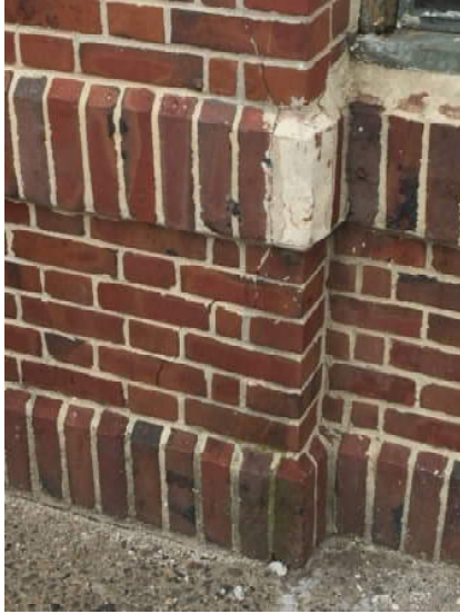
Photograph #11: Cracked front pier; implies rusting steel column within
