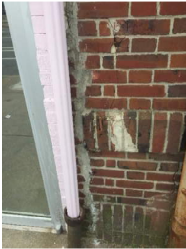
Photograph #3: NE Corner brick cracks
