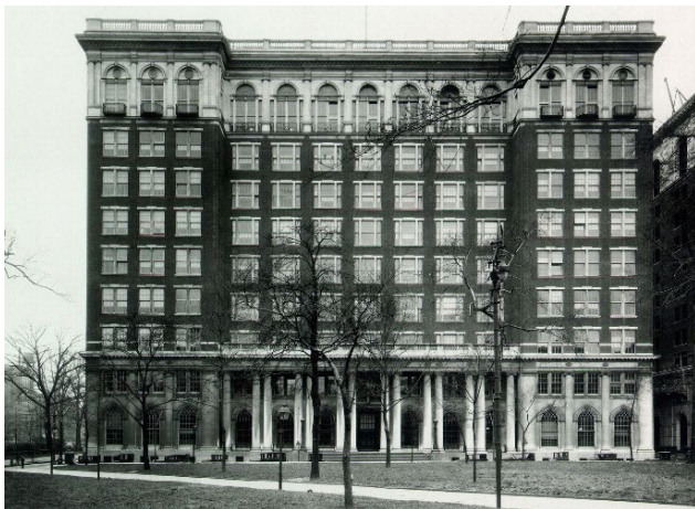
Curtis Publishing offices and printing plant, 1910
