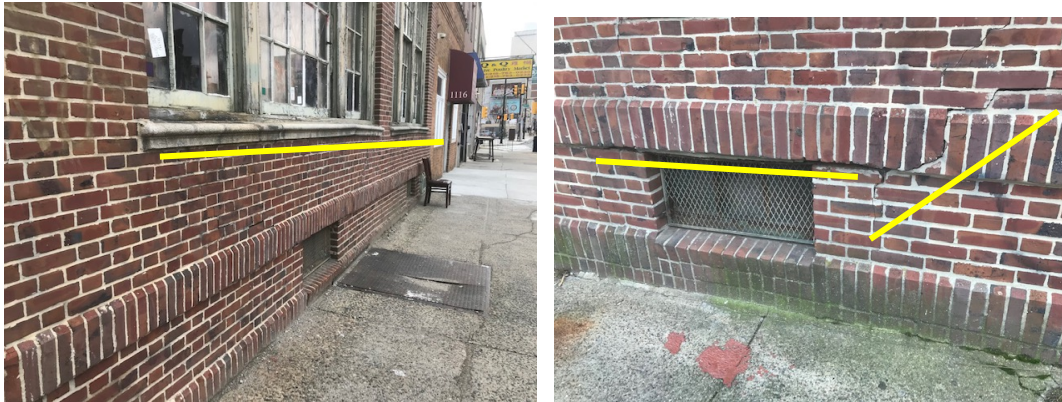
Façade looking west showing sills raised out of position and major cracking of spandrels caused by rust jacking of the basement windows
