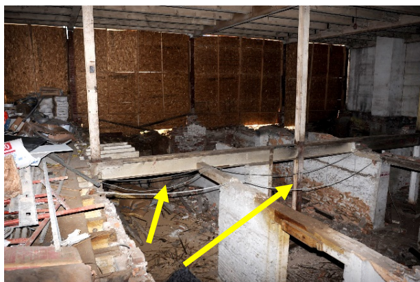
Rubble masonry party walls of original rowhouses; rubble masonry foundations of party walls and front wall (yellow arrows) from original rowhouses.
