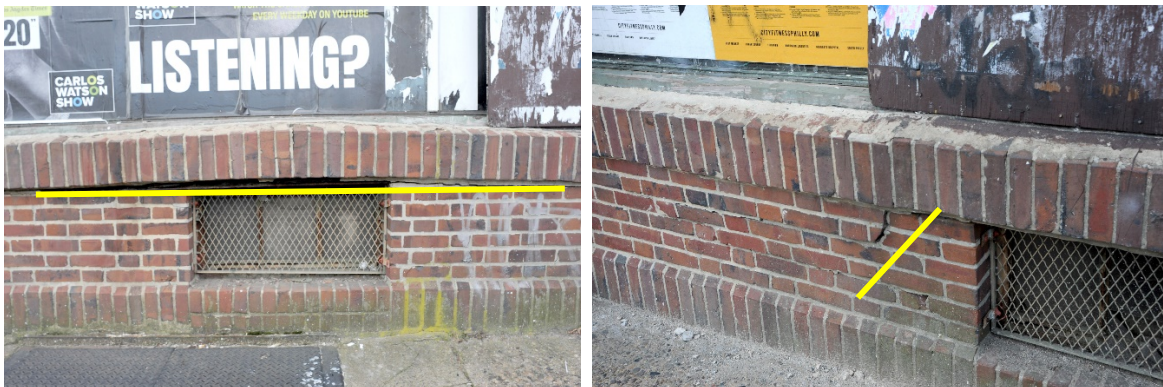
Left: steel lintel above window jacked out of position; right: soldier course pushed out of plane to left of window
