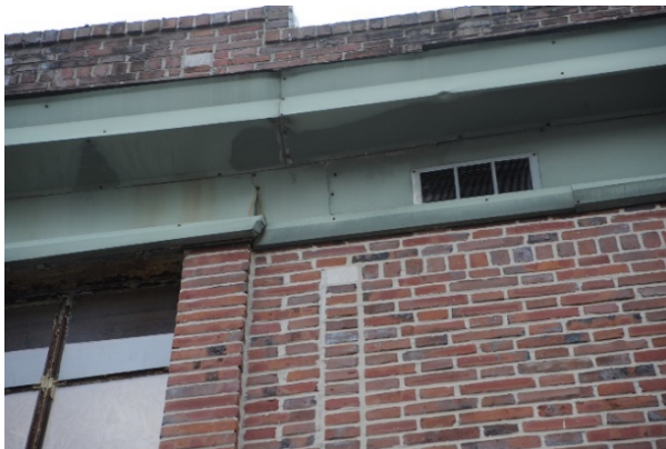
Left: sheet copper cornice (not stone) riveted together; end of copper cornice showing torn end where drain line removed – obviously metal. Not stone.
