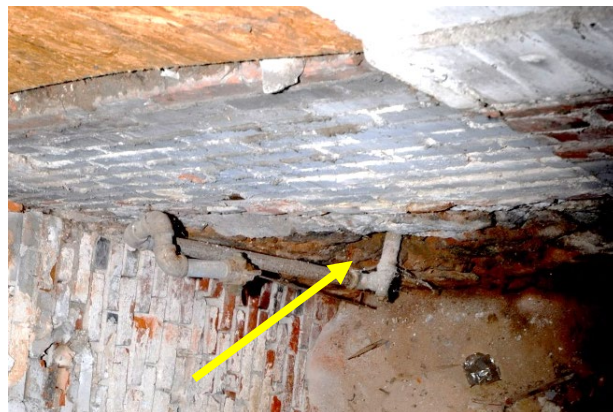
Rubble masonry party walls of original rowhouses; rubble masonry foundations of party walls and front wall (yellow arrows) from original rowhouses.
