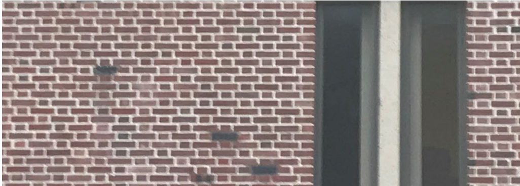
Flemish bond brick panels University of Pennsylvania Chemistry Building, Ballinger Co. and H2L2, 1969-73
