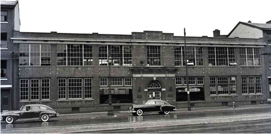
1106-14 Spring Garden in 1949; window sills flat, no distortion or evidence of obvious problems (Free Library of Philadelphia)
