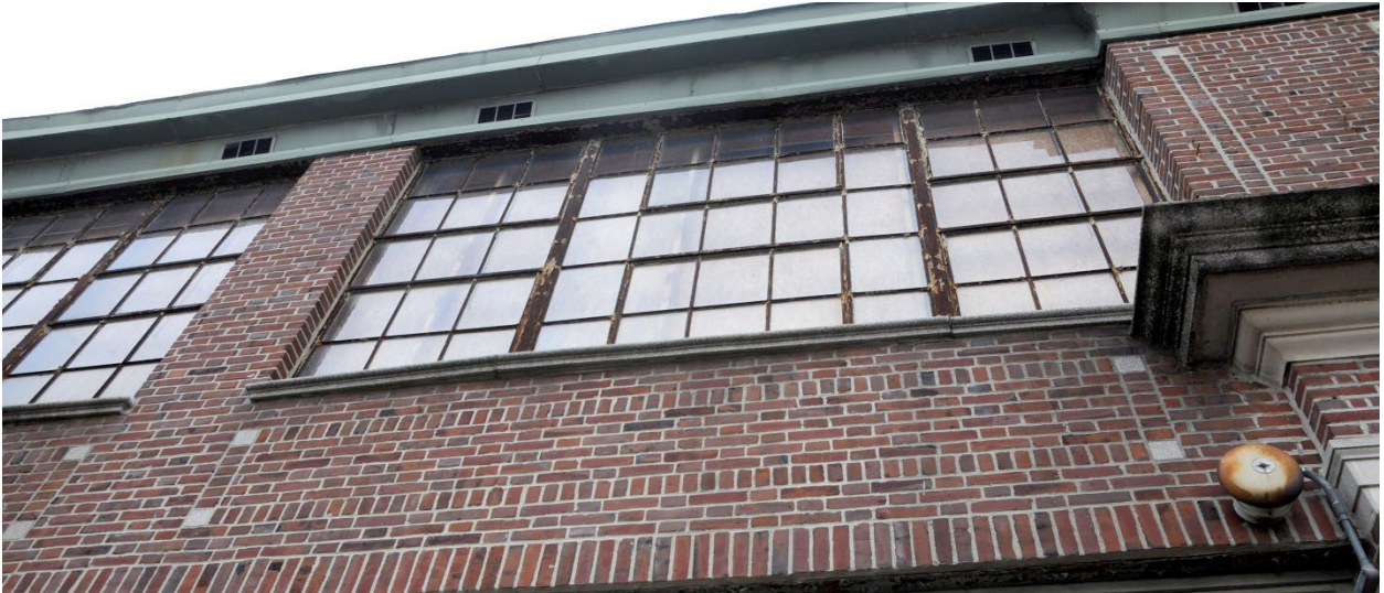
Copper cornice, banks of industrial sash, moderne paneling, soldier course brick spanning window openings – none of these features are Colonial Revival
