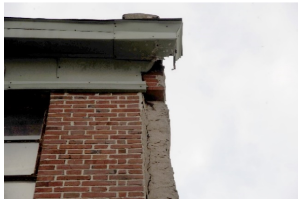
Left: sheet copper cornice (not stone) riveted together; end of copper cornice showing torn end where drain line removed – obviously metal. Not stone.
