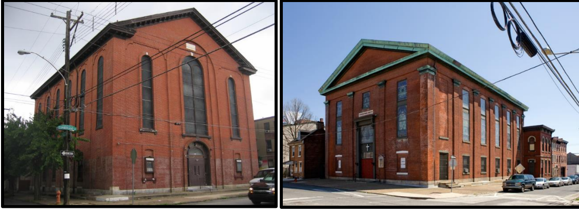
Figure 29. Left: The subject building is built on a commonly known form and plan, while also being a beautiful example of the Italianate style. Source: Flickr. Figure 30. Right: “Old Brick” is a Methodist Episcopal Church on Richmond Street in the Fishtown neighborhood near the Delaware River waterfront. While of the Greek Revival style, the building form is similar to the subject property. Source: Hidden City Philadelphia.
