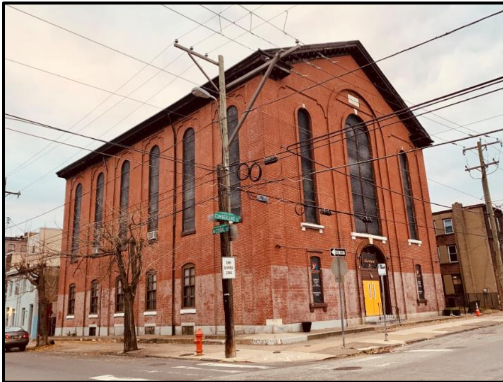
Figure 1. The side (east) and primary (north) elevations of the subject property. Source: Oscar Beisert, 2019.
