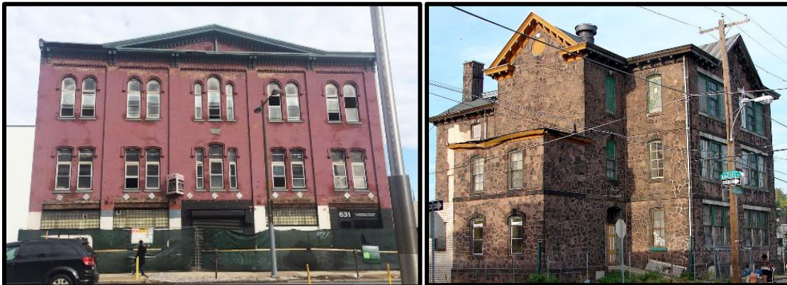
Figure 22. Left: The Thomas Hart Stable, N. Broad Street, Philadelphia (extant) was designed in the Italianate style and, like the subject property features a bracketed pediment, full arch top windows, and subdued pilasters, almost all of which is articulated in red brick. Source: Curbed Philly. Figure 23. Right: The David Farragut School (1873), West Kensington, Philadelphia is an Italianate style school at 170 W. Cumberland Street, built at the same time as the subject property. Source: https://en.wikipedia.org/wiki/David_Farragut_School_(Philadelphia,_Pennsylvania) .
