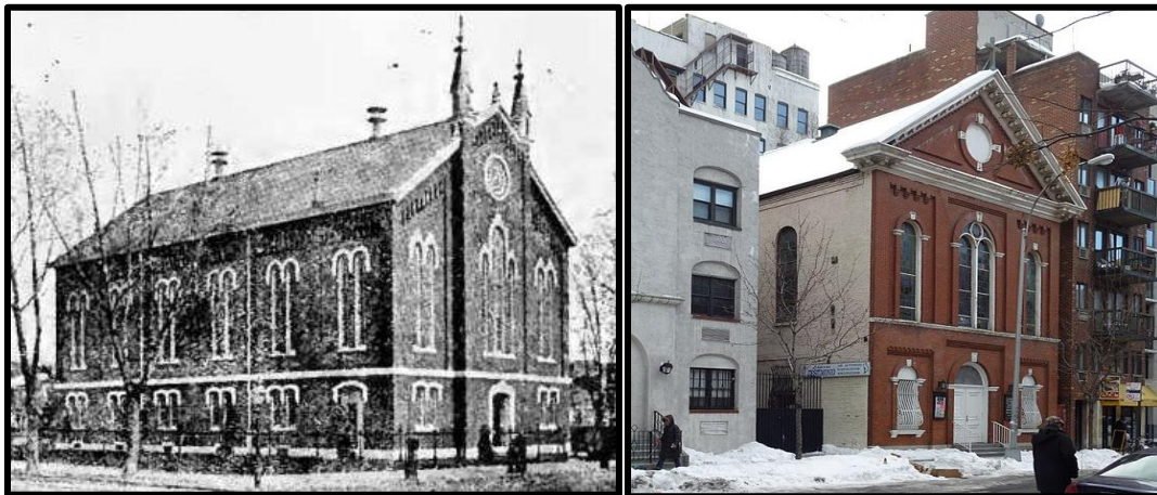
Figure 20. Left: The First Methodist Episcopal Church of Camden was built on the same form and also influenced by the Italianate style. Source: dvrbs.com. Figure 21. Right: St. Benedict the Moor Church (1869), 342 West 53 rd Street, Hell’s Kitchen, Manhattan, New York City was designed in the Italianate style for an African American congregation. Source: https://www.revolvy.com/page/St.-Benedict-the-Moor-Church-(New-York-City) .
