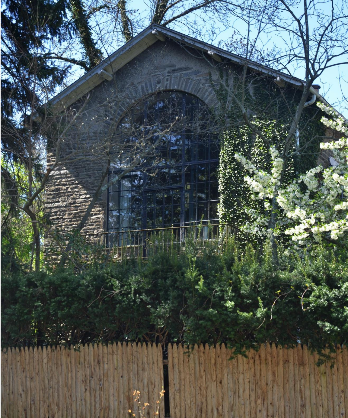
Figure 6: Northeast side elevation, rear addition detail.
