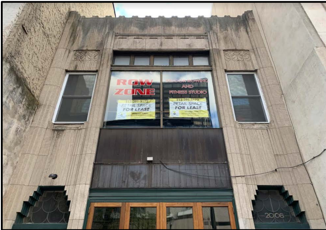
Figure 3. The primary (north) elevation of the subject property. Source: Oscar Beisert, 2020.
