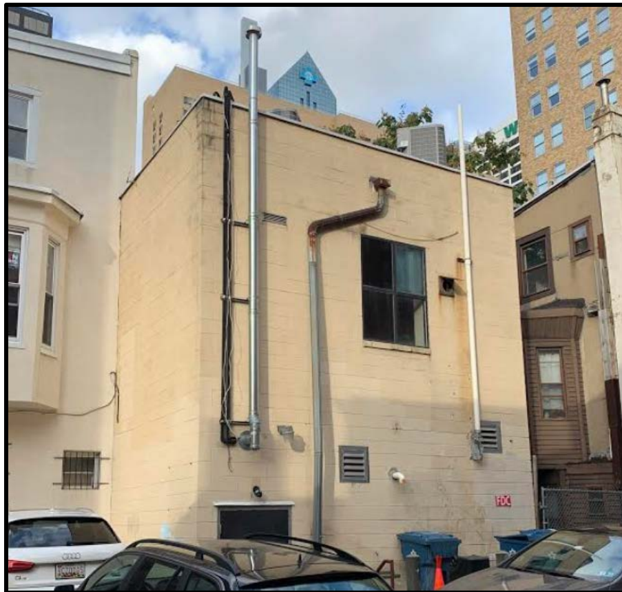
Figure 7. The rear (south) elevation of the subject building. Source: Oscar Beisert, 2020.
