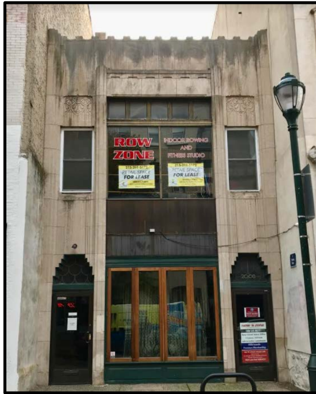
Figure 1. The primary (north) elevation of the subject property. Source: Tim Kerner, 2020.
