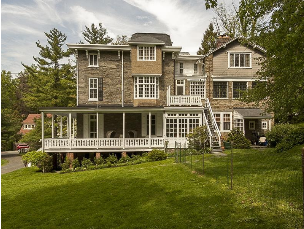
Figure 7: Southwest side elevation, c. 2014.
