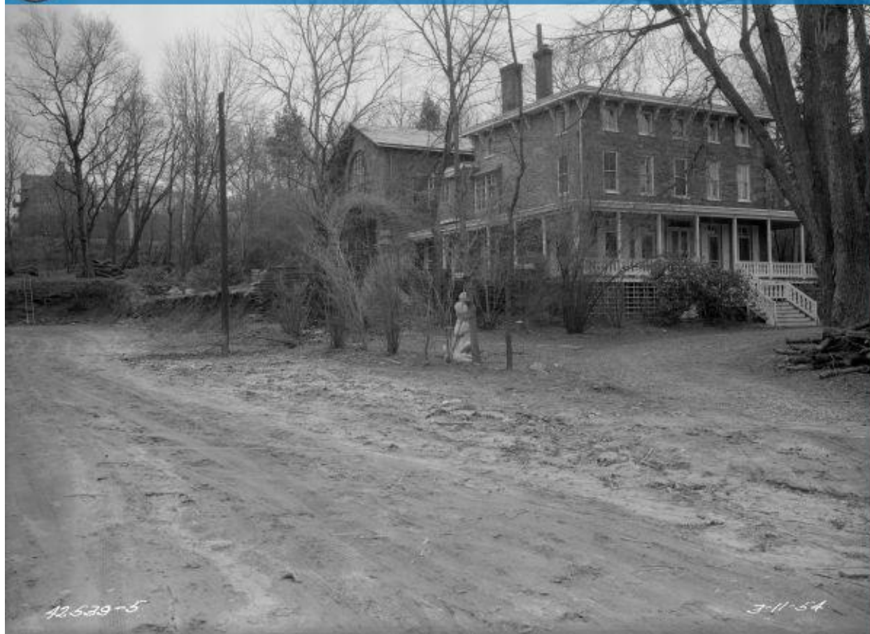
Figure 9: Property in 1954 during widening of Crefeld Street. Photo via PhilaHistory.org.
