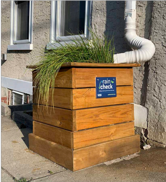
The Philadelphia Water Department provides rain barrels to divert water from roof downspouts from storm water drains into storage containers that can be used to water plants and gardens.
