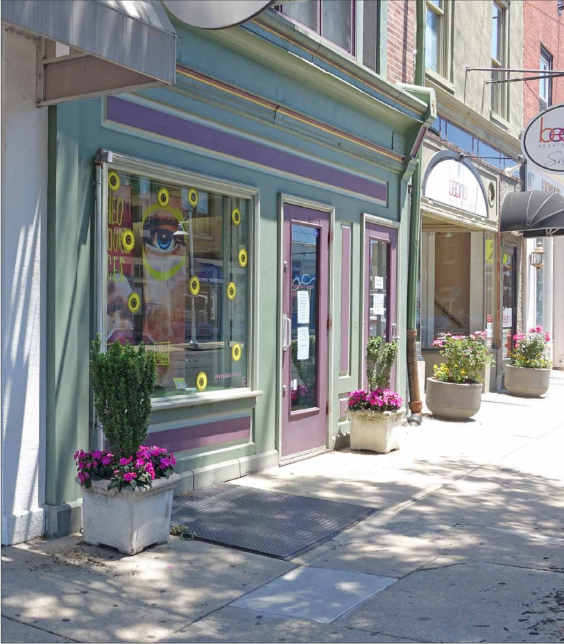
Although many of the commercial buildings on Main Street are brick, wood storefronts, like wood framed houses, are poor candidates for dry floodproofing.
