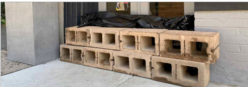
Although barriers such as sandbags may reduce floodwater from entering a building, they do not comply with Philadelphia floodplain regulations.
