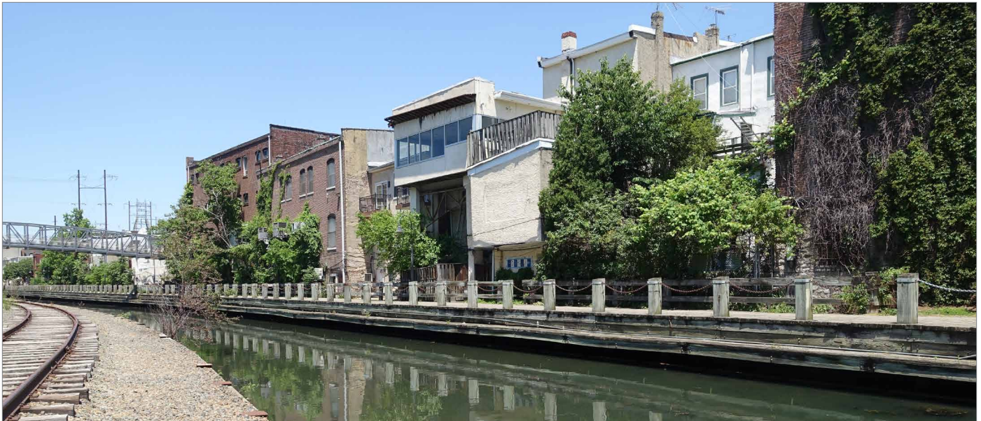
Rear portions of buildings on Main Street are at lower elevations and would particularly benefit from regular, consistent maintenance.
