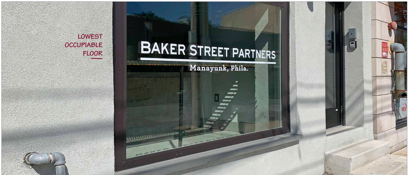
The first floor of this office has been raised at the interior of the building, while maintaining the height of the door and storefront window.
