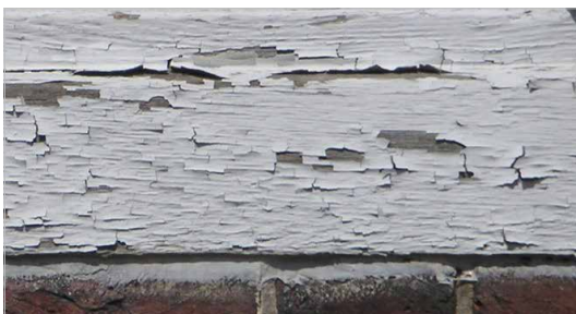
Open joints around windows and door frames can provide a path for water infiltration. Regular replacement of sealant is required for it to retain its effectiveness to prevent water infiltration.
