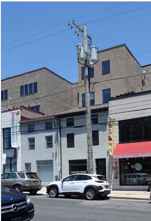
The loss or limiting of first floors may cause some property owners to consider an elevated addition to recapture lost square footage. In this example, the addition is set back from the street with the intent of limiting visibility.
