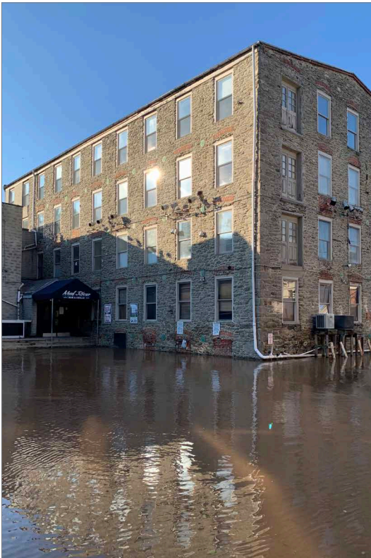
Exposure to floodwater can be detrimental to historic buildings and features.
