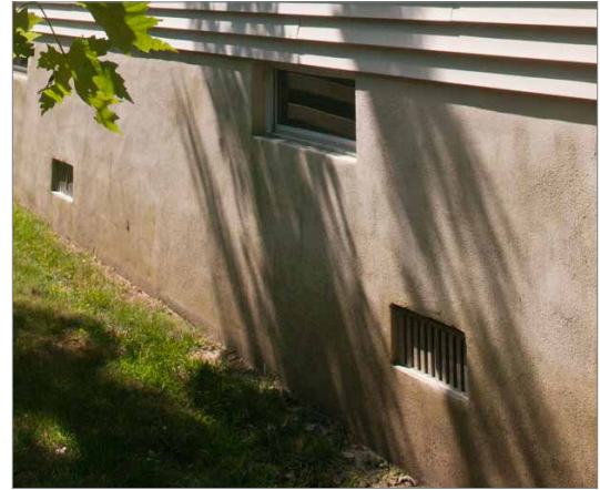
Flood vents, such as those located along the foundation, allow the free passage of water in and out of a closed foundation or building.
