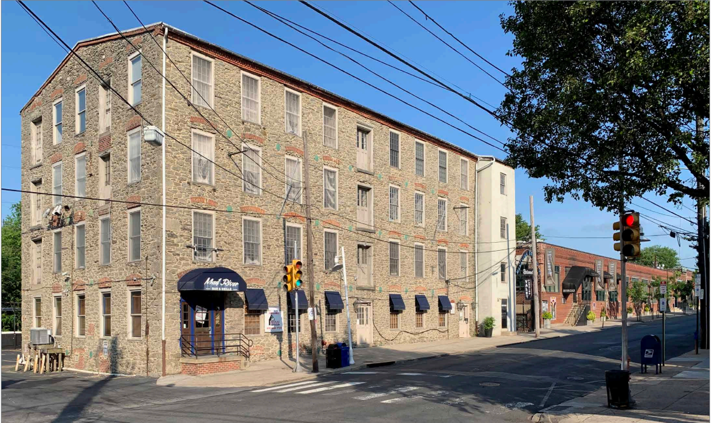
Main Street slopes down to a low point near Shurs Lane. Properties close to the corner are some of the most vulnerable in the Manayunk Main Street Historic District. The Manayunk Brewing Company, located in the lower level of the red brick building, has been significantly flooded several times.
