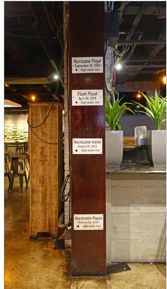
Floodwater heights from past flood events are marked inside the Manayunk Brewing Company. Three of the four markers identify hurricane-related flooding.
