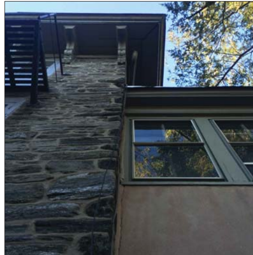
9. Detail of connection of porch addition to historic building at second story (east facade).
