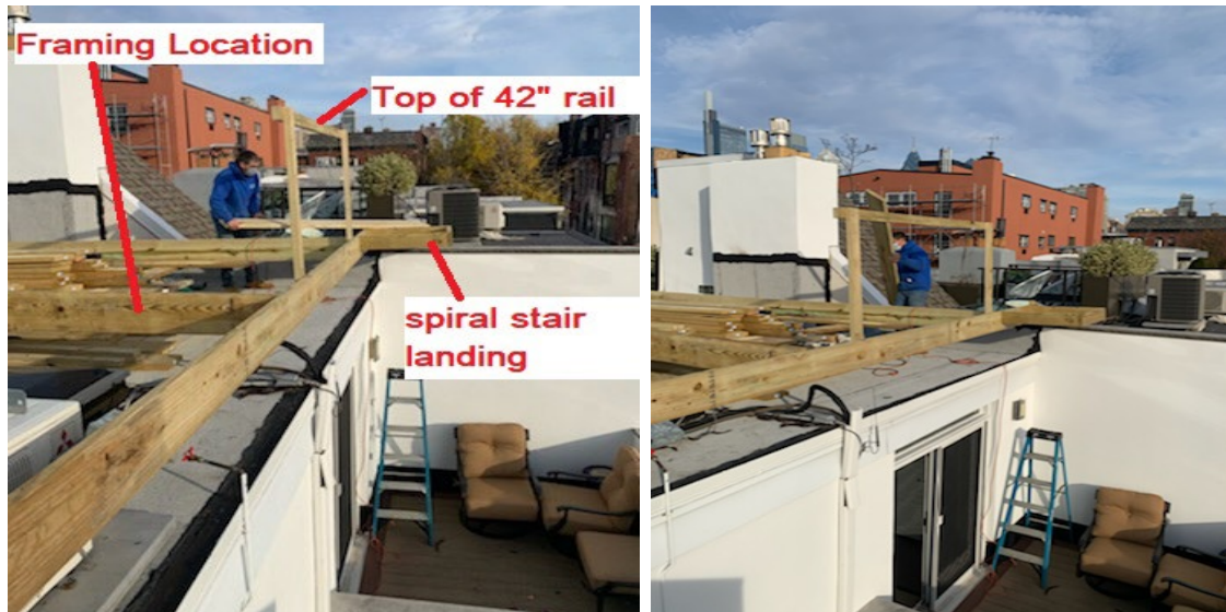
Proposed framing / railing location at front of building.
