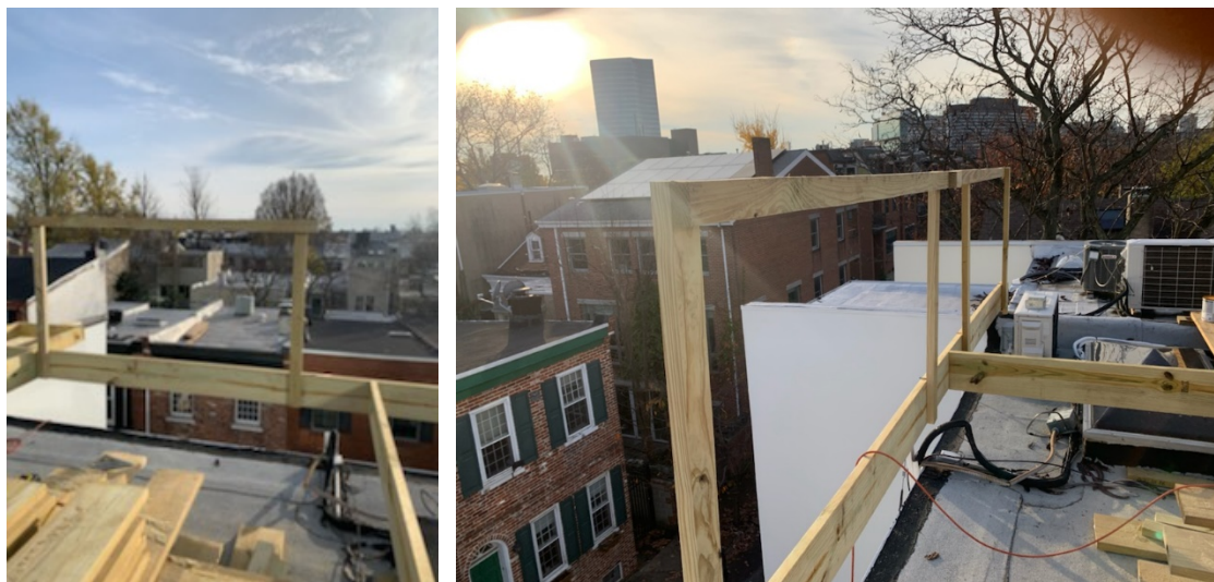
Proposed railing view at front of building from rooftop surface. Railing to be 42" from deck surface to top rail.
