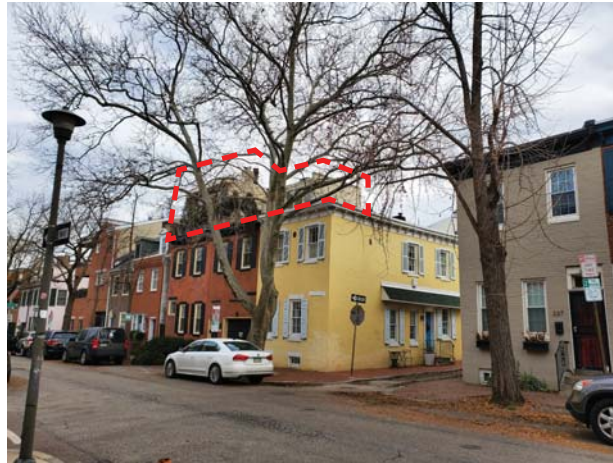
7 View from sidewalk looking northeast at the third floor addition to 331 S 25th St
