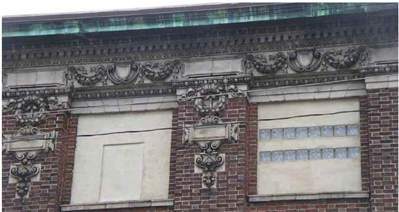
Infilled windows at third floor of 1902 building, showing high level of ornamentation.
