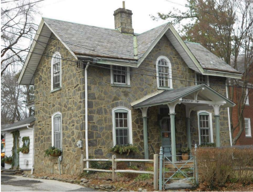
Figure 4 - 3/4 southwest facing view of subject property. Nancy Pontone, February 2020.
