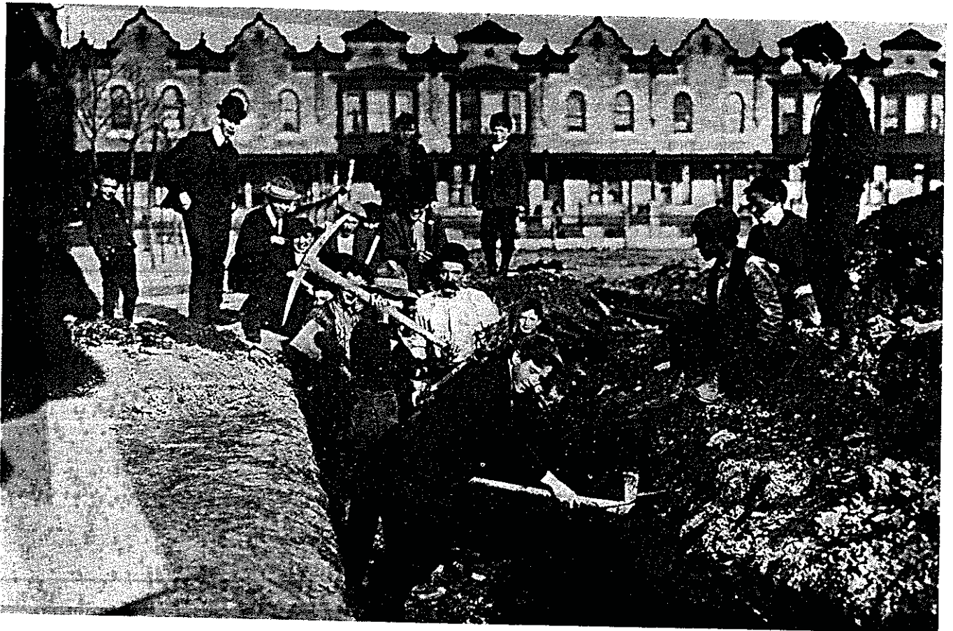
ANOTHER PICTURE OF THE WORK ON THE FOUNDATION, APRIL, 1902
