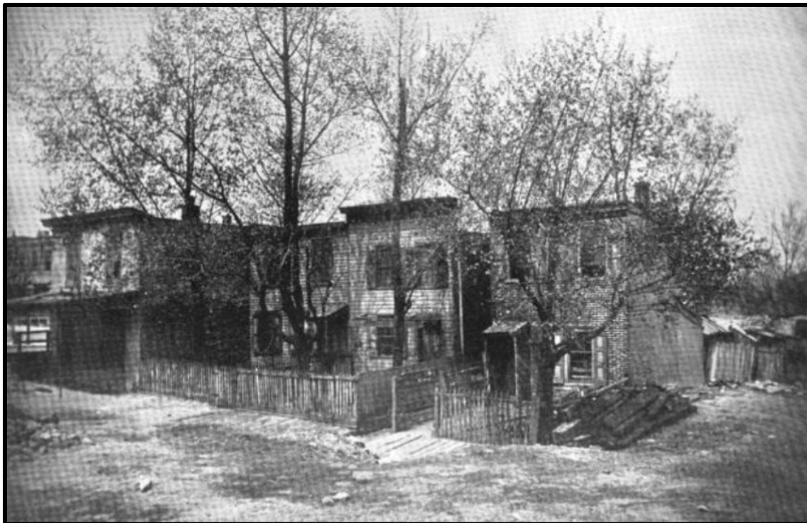
Figure 11. Four frame dwellings at “Laniganville, near Thirty-Eighth and Poplar Streets” just before demolition c1903 ( West Philadelphia Illustrated [1903]). This figure shows other examples of frame dwellings that once characterized the early built environment of West Philadelphia.
