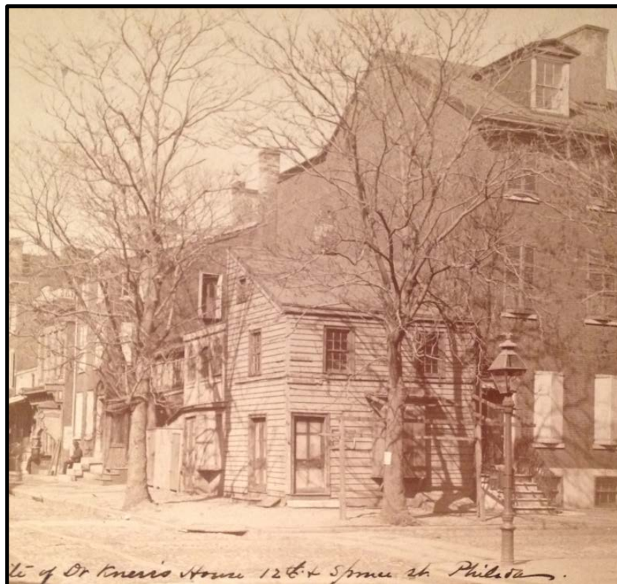
Wooden House at the Corner of 12 th and Spruce. Source: The Historical Society of Pennsylvania.
