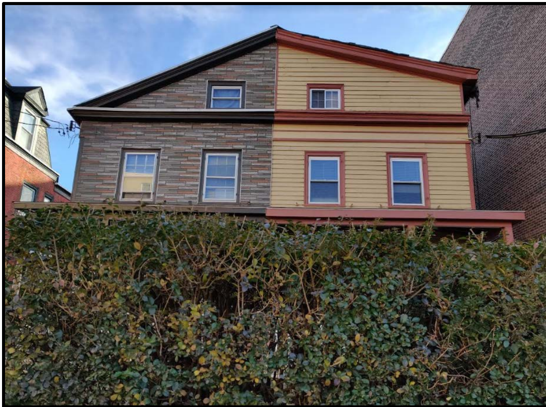
Figure 4. Left: Looking south at the subject property's primary (northeast), and northwest elevations.
