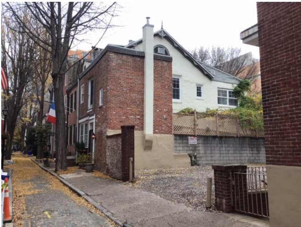
253 Quince Street as viewed from the south end of the 200 block
