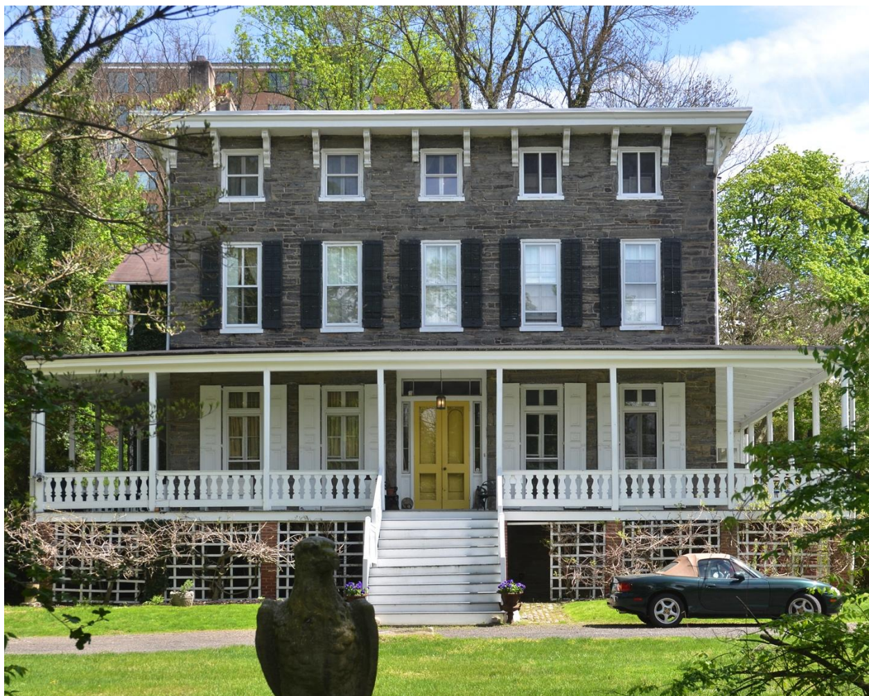
Figure 1: Primary northwest elevation facing Rex Avenue.
