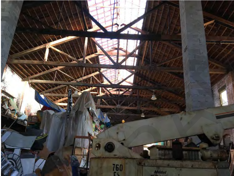
Figure 12 (Photo 9): View of Interior Skylight, Looking North
