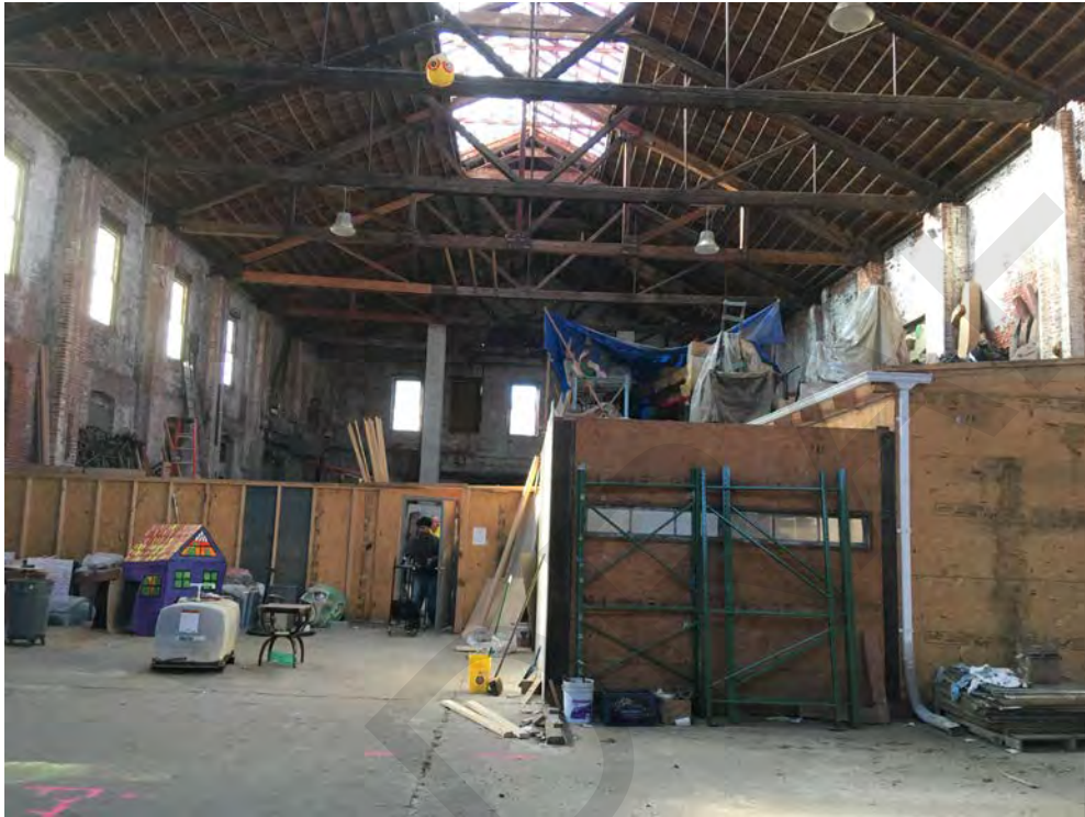
Figure 8 (Photo 7): View of Interior, Looking South
