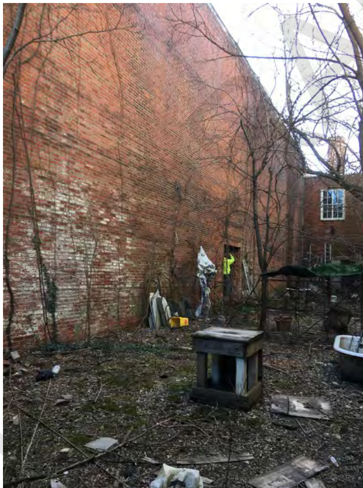
Figure 7 (Photo 6): View of West Elevation, Looking Southeast
