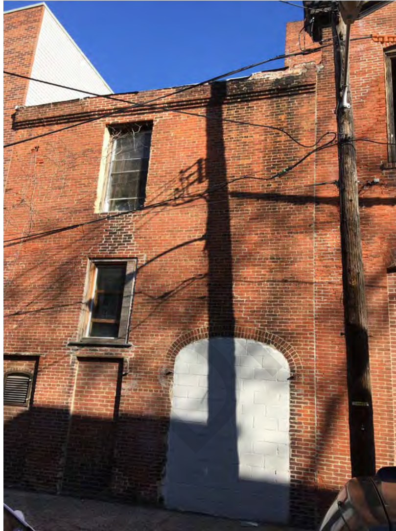
Figure 4 (Photo 3): View of c. 1885 Addition, Looking North
