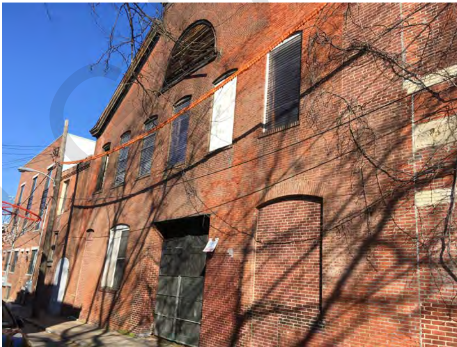
Figure 6 (Photo 5): View of South Elevation, Looking Northwest
