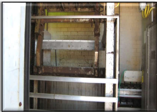
Figure 19: CIP Project: Installed East Influent Bar Rack at Influent Pumping Station
