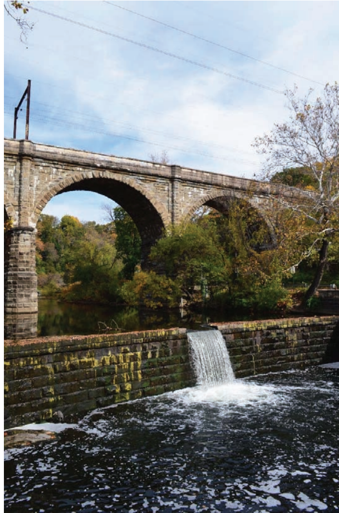
SEPTA bridge over Wissahickon Creek
