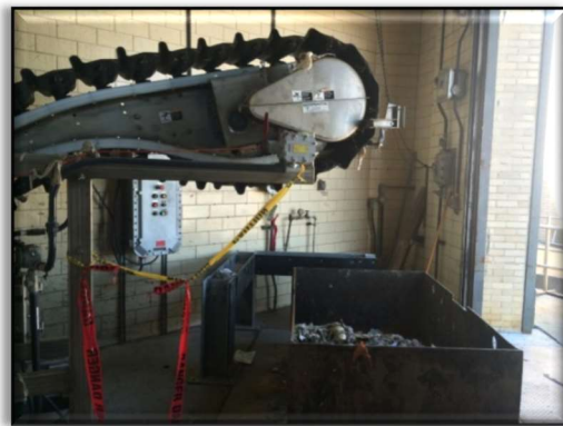
Figure 19: CIP Project: Installed East Influent Bar Rack at Influent Pumping Station
