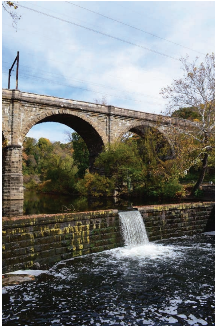
SEPTA bridge over Wissahickon Creek
