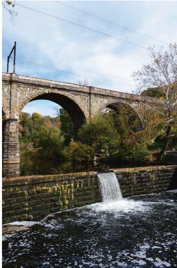
SEPTA bridge over Wissahickon Creek
