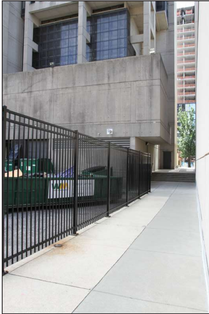
Figure 17: Looking south along the pedestrian passageway lining the west elevation and that connects Ludlow Street with the plaza. Note the gridded, double-skin, glass wall visible on the upper lower levels. These windows provide natural light to the interior atrium. (Source: Allec Davis, August 2019)
