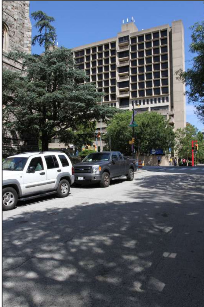
Figure 27: View of the south elevation of the International House, from 37th Street. (Source: Allee Davis, August 2019)
