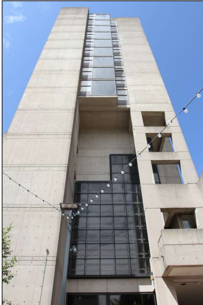
Figure 33: East elevation of the International House, from 37th Street. Note the gridded, double-skin, glass wall visible on the upper lower levels. These windows provide natural light to the interior atrium. (Source: Allee Davis, August 2019)
