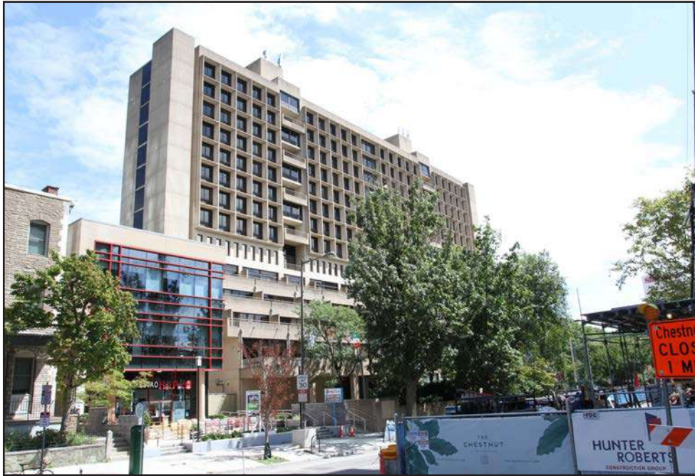
Figure 3 (top): View of the south elevation of the International House, from Chestnut Street. (Source: Allee Davis, August 2019)
