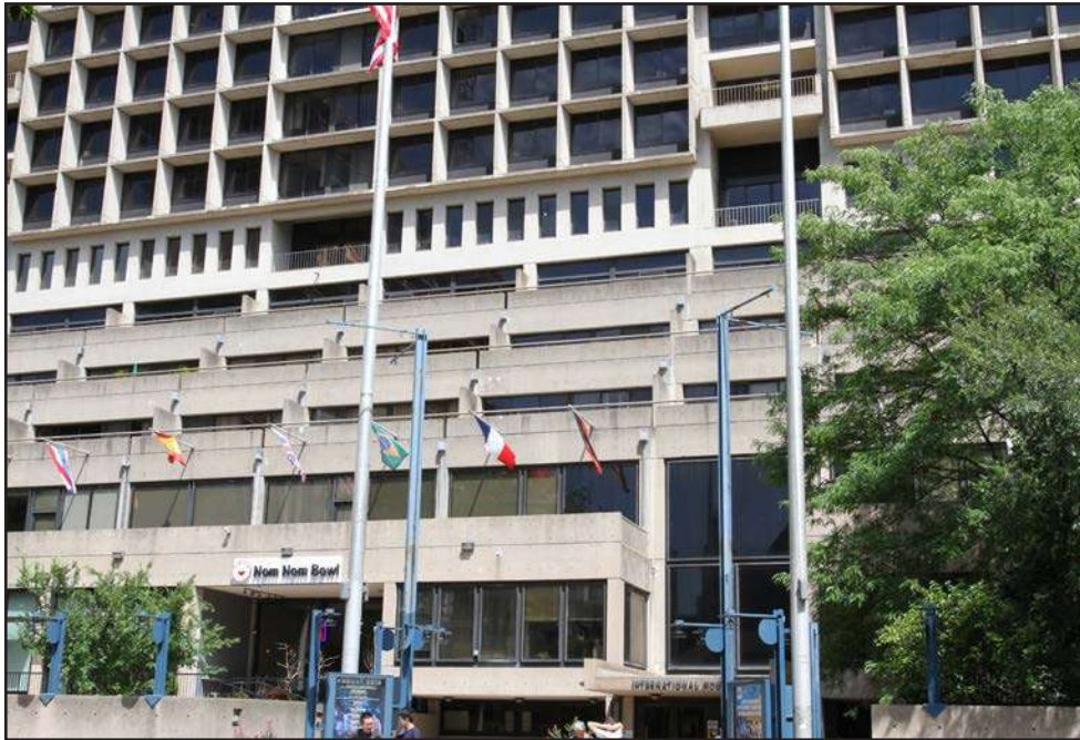
Figure 20 (top): View of the south elevation of the International House, from Chestnut Street. (Source: Allee Davis, August 2019)
