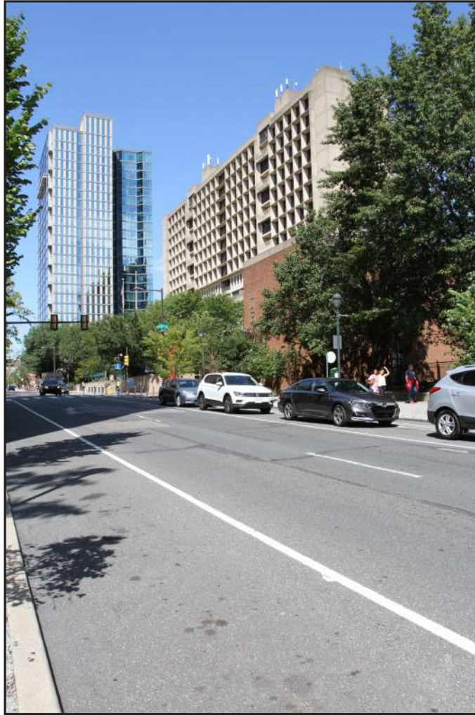
Figure 6: View of the south elevation of the International House, from Chestnut Street. (Source: Allee Davis, August 2019)
