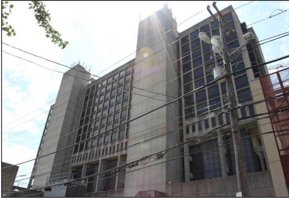
Figure 25 (top): View of the north elevation of the International House, from Ludlow Street. (Source: Allee Davis, August 2019)
