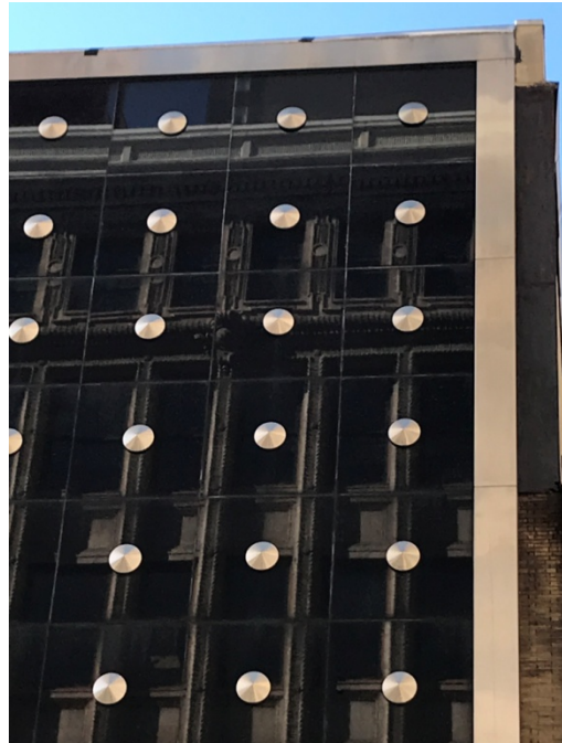
Image 7 (left): 1206 Chestnut Street, upper floors of façade, showing cladding in rows of polished black granite panels with stainless steel discs, September 2020 Image 8 (right): 1206 Chestnut Street, detail of polished black granite panels with stainless steel discs and stainless steel band trim, September 2020
