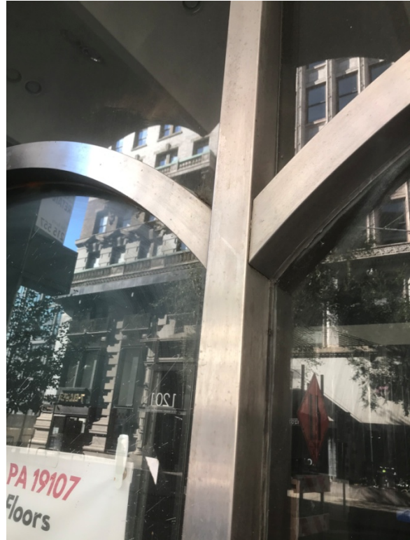
Image 5 (left): 1206 Chestnut Street, showing recessed entrance extant original clock and glass wall with stainless steel mullions, September 2020 Image 6 (right): 1206 Chestnut Street, stainless steel mullion joint detail, September 2020
