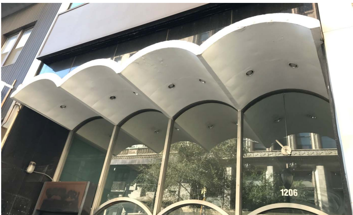
Image 4: 1206 Chestnut Street, concrete canopy detail, September 2020
