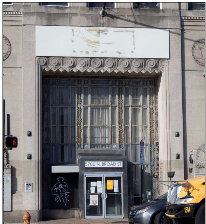
Figure 3: Entrance to 5700 North Broad Street. Photograph by Adrian Trevisan, 2020.
