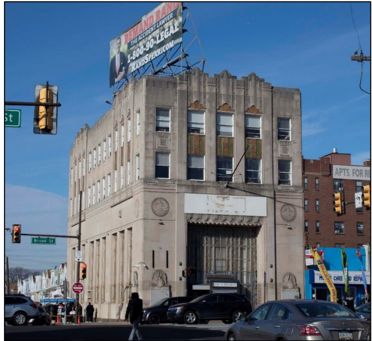
Figure 2: 5700 North Broad Street. Photograph by Adrian Trevisan, 2020..
