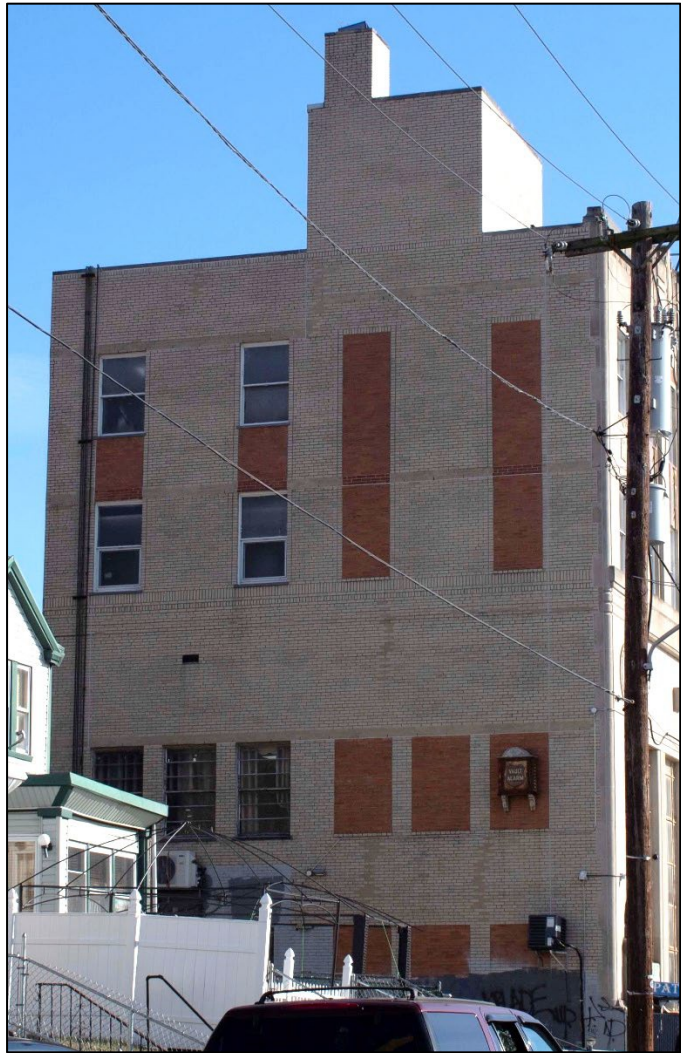
Figure 8 Rear, West, facade. Photograph by Adrian Trevisan, 2020.
