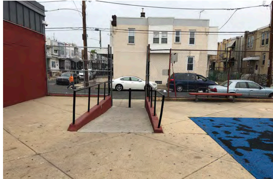
Entry ramp does not meet code
