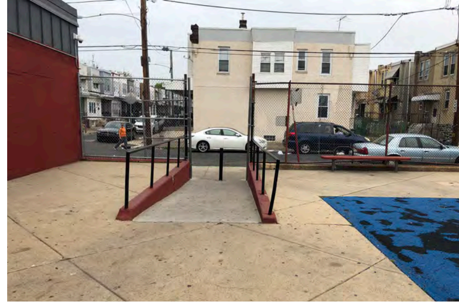
Entry ramp does not meet code
