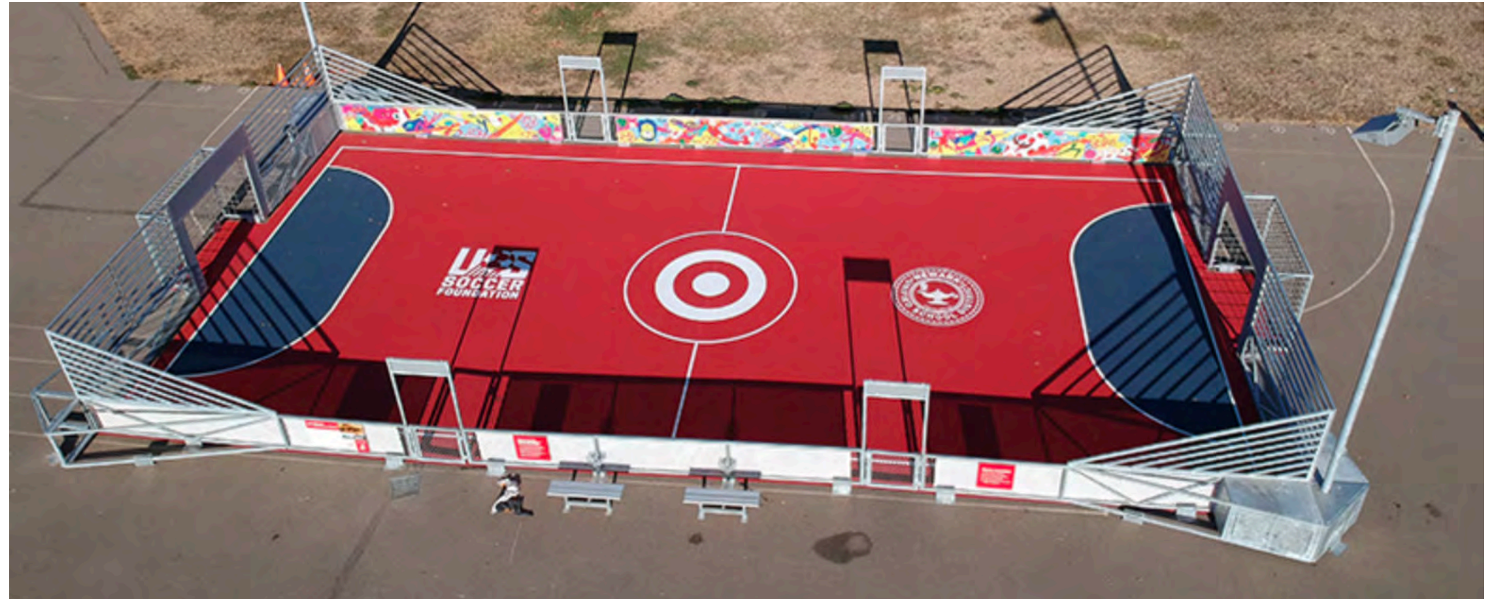
Former hockey court at back of site will be turned in to a soccer mini-pitch. The mini-pitch system will have surrounding low metal walls, entry gates, and goals as shown.
