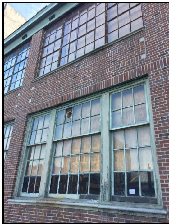
Looking southeast, an eastern bay of the primary elevation showing the windows at the first and second floors. Source: Andrew Palewski.
