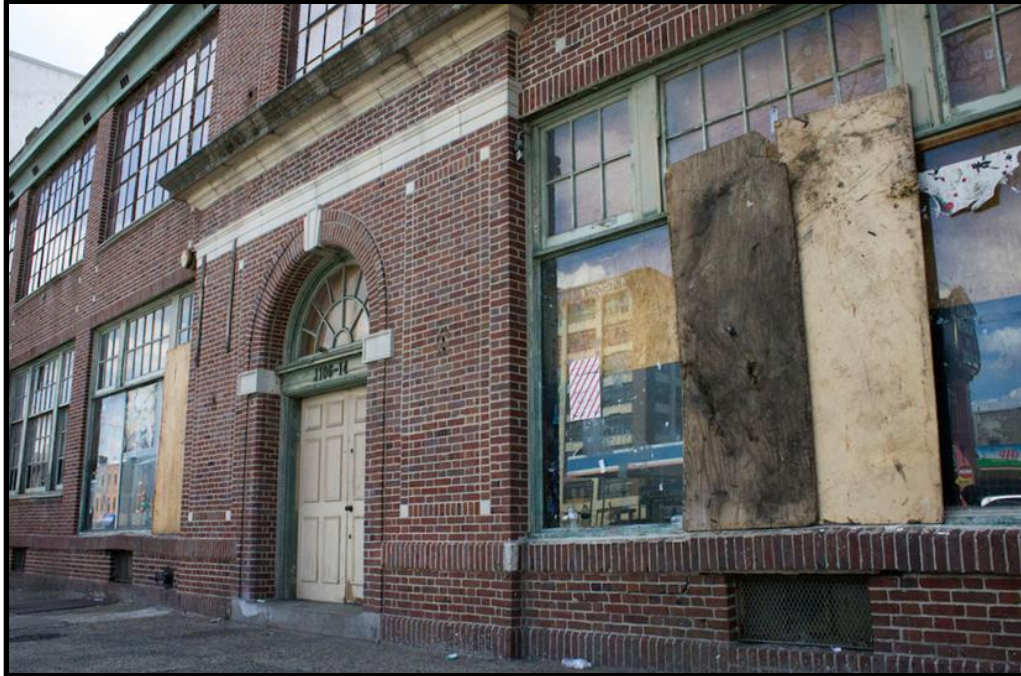
Looking southeast, the central bay of the subject property. Note the brickwork, the stone or concrete details, and the original windows. Source: Michael Bixler.
