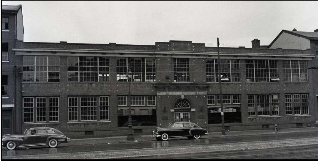
Looking south at the primary elevation of the subject building in c. 1949, during the last years of Woodland Wanger Co.'s use of the building. Source: the Free Library of Philadelphia.
