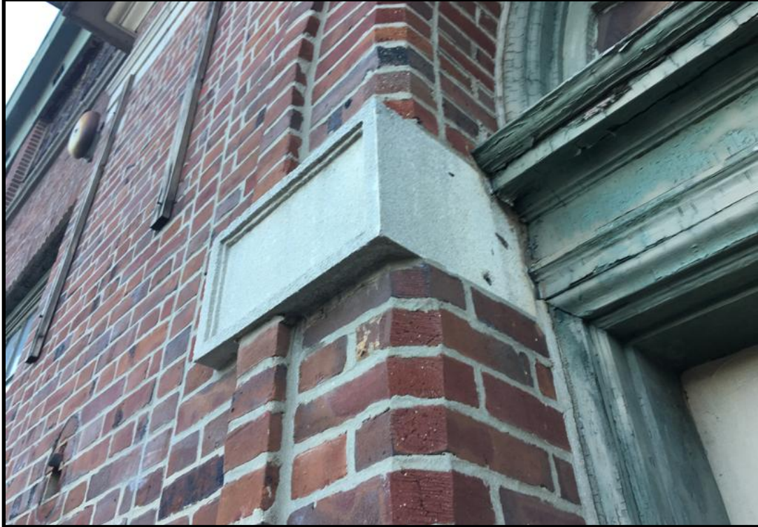
Detail photograph of key block within the central bay and the door surround of the primary entrance. Source: Andrew Palewski.
