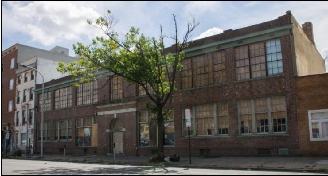
The Woodward-Wanger Building, later known as the Lawsonia Building, 1106-1114 Spring Garden Street. Source: Michael Bixler.
