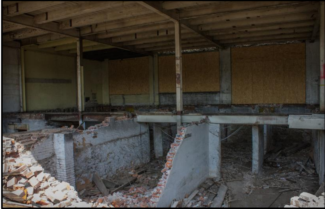
Looking northwest at the rear and interior of the subject building. Source: Michael Bixler.
