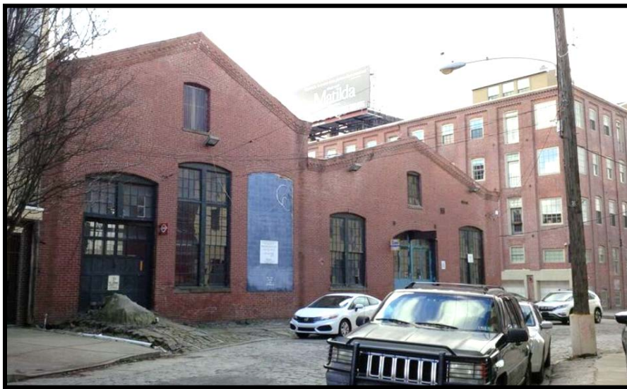
Figure 5: The primary (north) elevations of Building 10. The portion of the building on the left of the image will be referred to as the eastern block, while the portion on the right of the image will be referred to as the western block. Source: Michelle Shuman, 2018.
