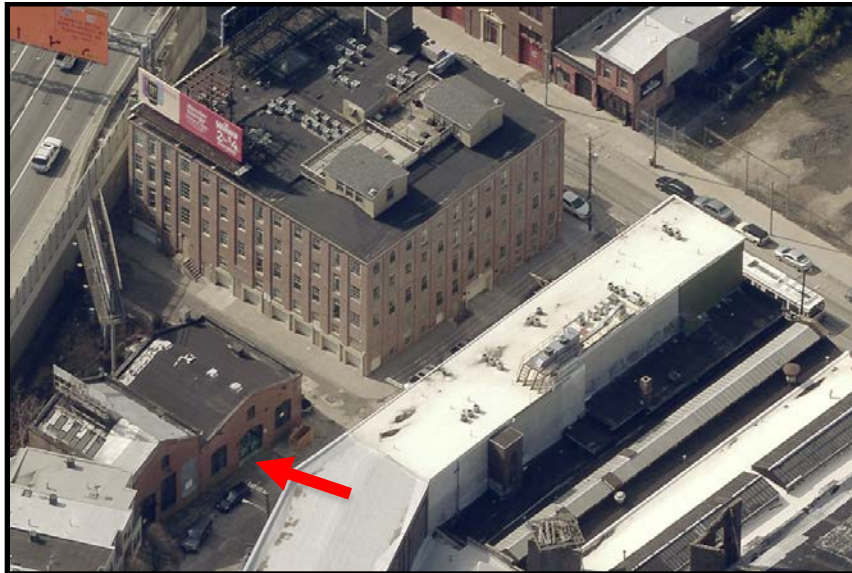
Figure 2: Looking southwest towards the primary (north) elevation of the subject property within the context of the former Elevator Works. Source: Atlas, City of Philadelphia, 2018.
