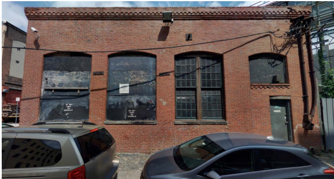
Figure 11: West, Sarah Street elevation. Source: Cyclomedia, 2018.
