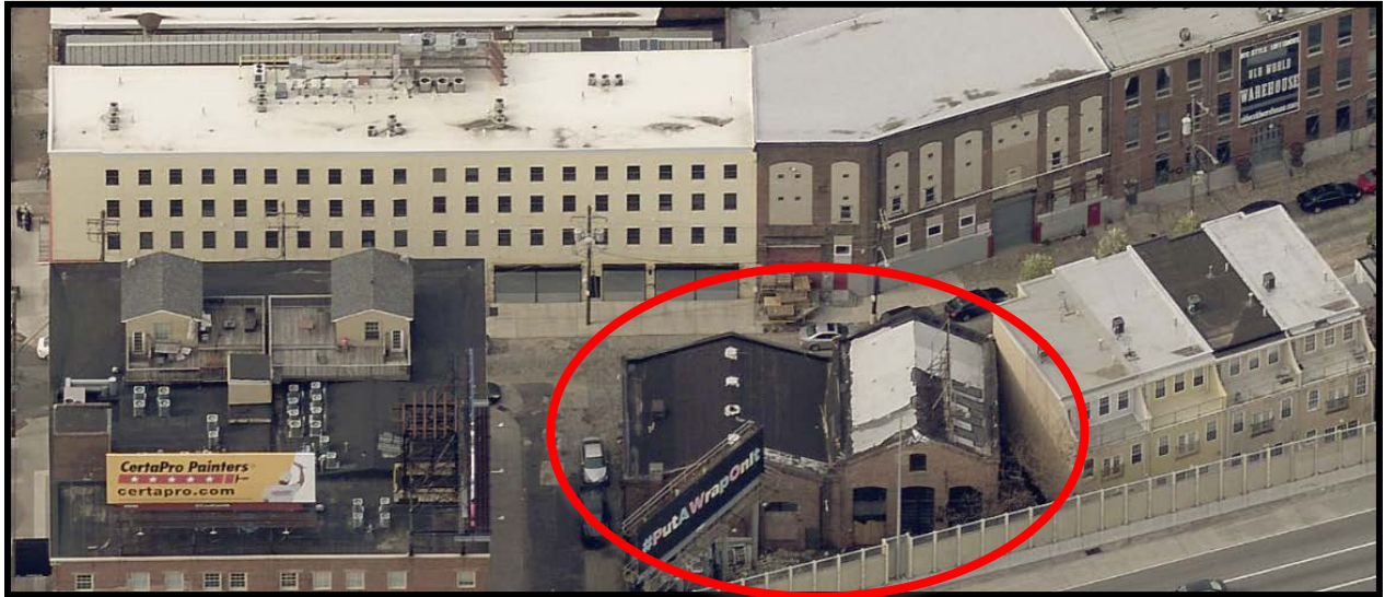
Figure 14: Looking north at the rear (south) elevation of the subject property within the context of the former Elevator Works. Source: Atlas, City of Philadelphia, 2018.
