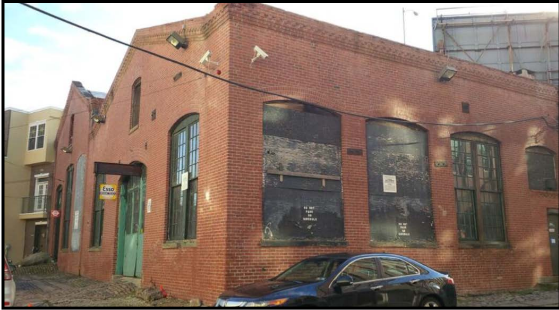
Figure 10: The primary (north) and west elevations of the western block of Building 10, from the corner of Wildey and Sarah Streets. Source: Michelle Shuman, 2018.
