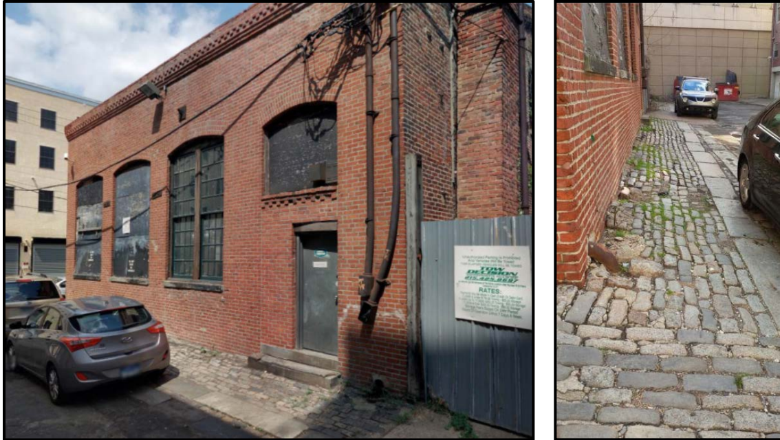
Figure 12: Details of the west, Sarah Street elevation and paving.
