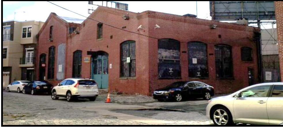
Figure 4: The primary (north) and side (west) elevations of Building 10. Source: Michelle Shuman, 2018.
