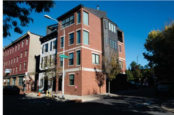
5 - View of 215-217 Vine Street, Looking Northwest
