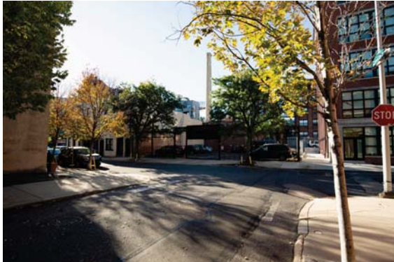
4 - View of 214-220 Vine Street, Looking South from N. American St
