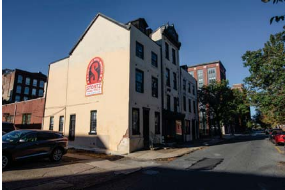
1 - View of 208-220 Vine Street, Looking West
