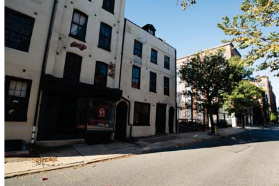
2 - View of 210-220 Vine Street, Looking West
