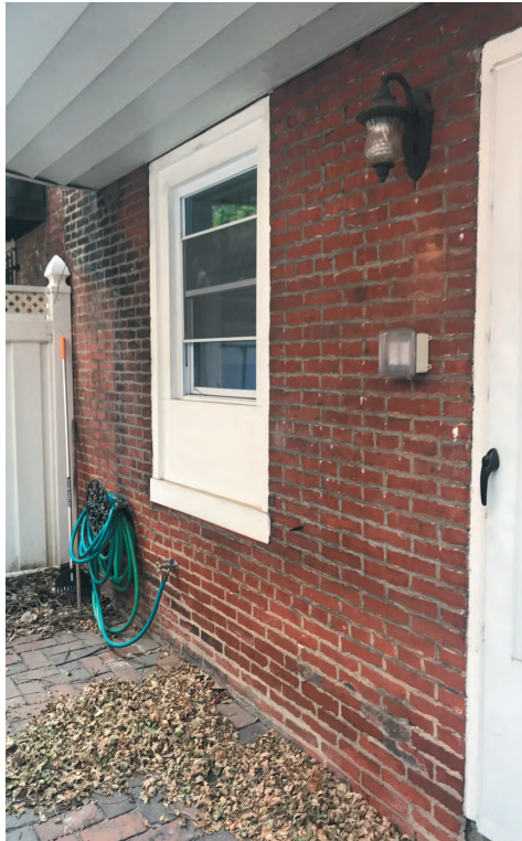
smaller window in masonry opening / siding covering bottom of bay
