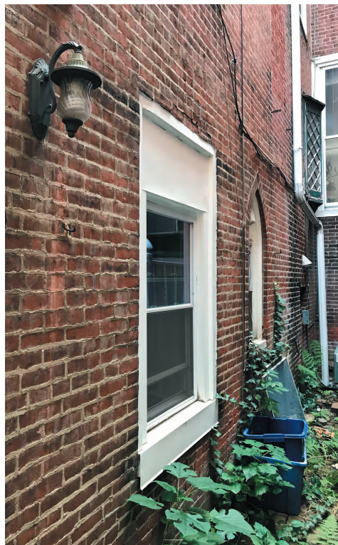
smaller window in masonry opening
