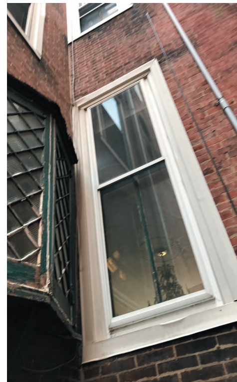
accent window / aluminum cladding on window frame and sill/ storm window
