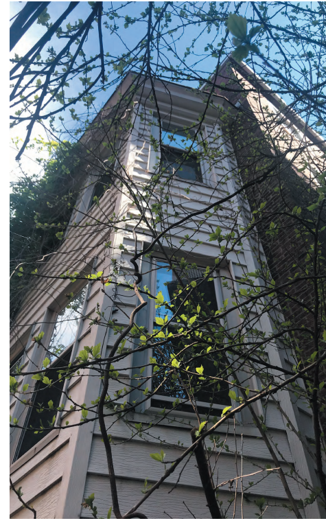
siding clad bay / aluminum cladding on window frame and sill/ storm window
