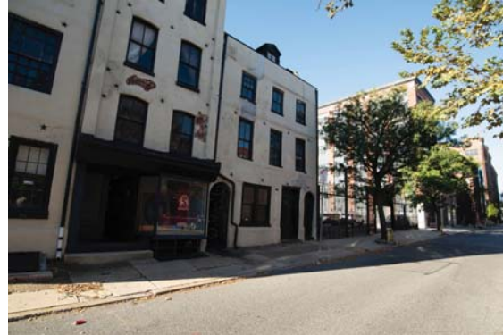
2 - View of 210-220 Vine Street, Looking West
