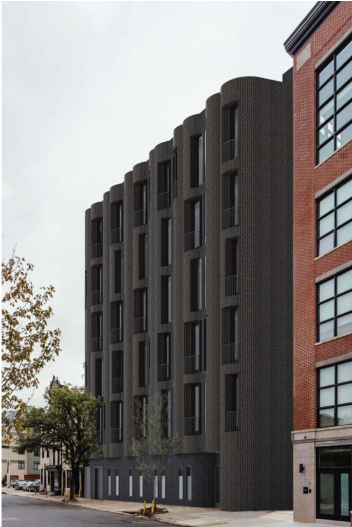
VIEW FROM VINE ST. LOOKING EAST
