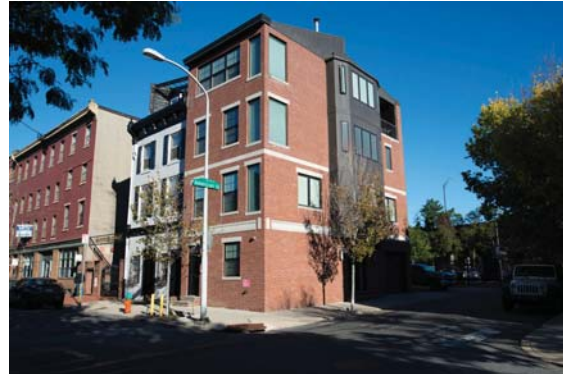
5 - View of 215-217 Vine Street, Looking Northwest
