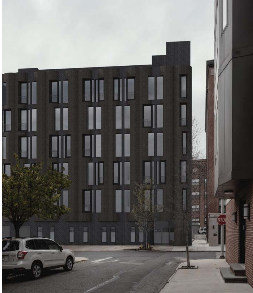
VIEW FROM N AMERICAN ST. LOOKING SOUTH
