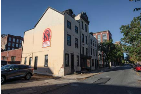
1 - View of 208-220 Vine Street, Looking West
