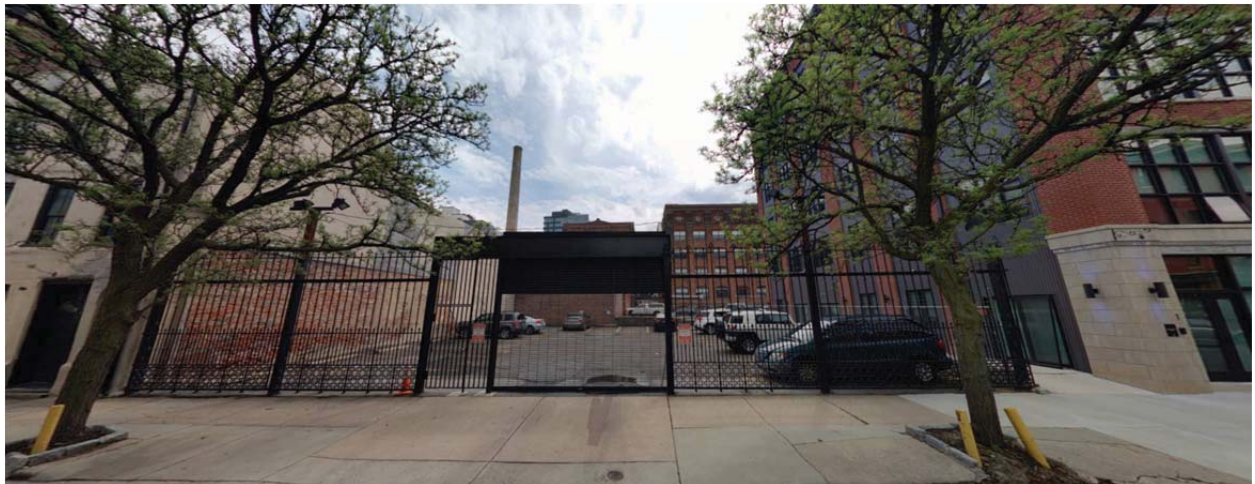
Figure 2: The parking lot and non-historic fencing at 214-20 Vine Street, May 2020. Source: Cyclomedia.
