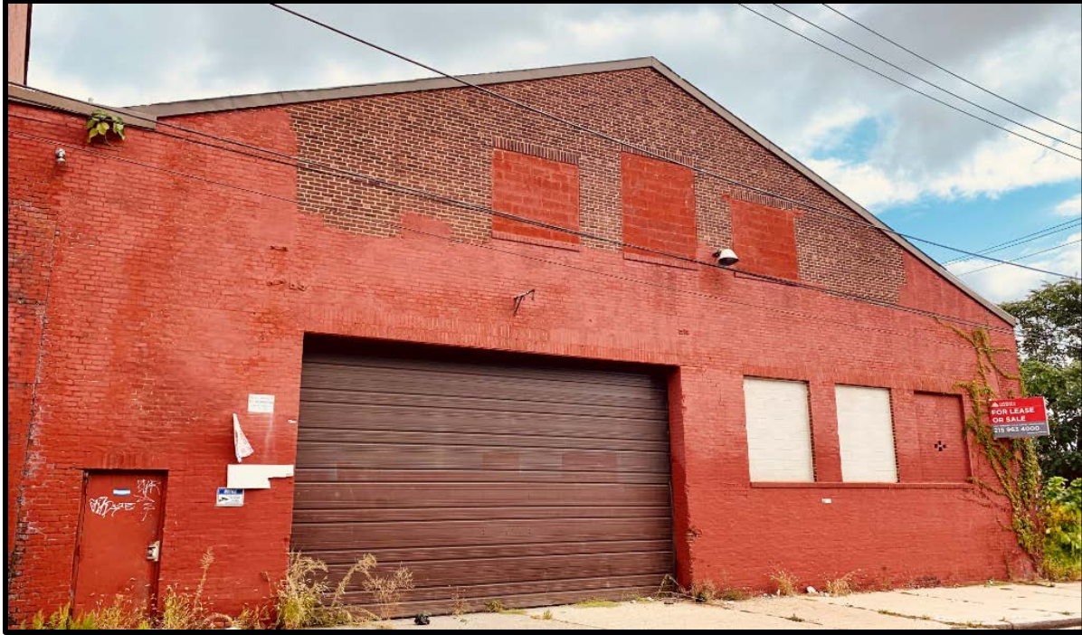
Figure 20. The south elevation of Building 3. Source: Oscar Beisert, 2019.
