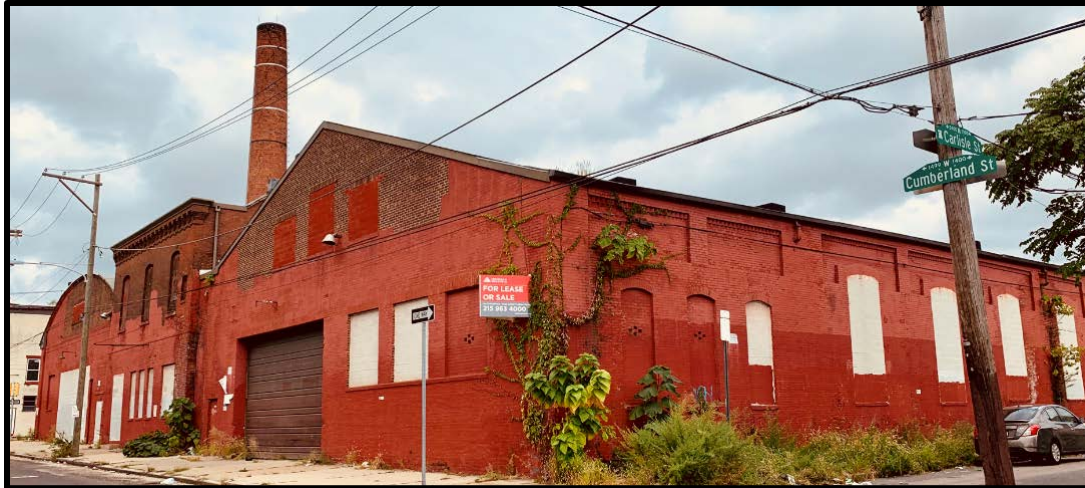
Figure 18. The south and east elevations of Buildings 1 and 3. Source: Oscar Beisert, 2019.
