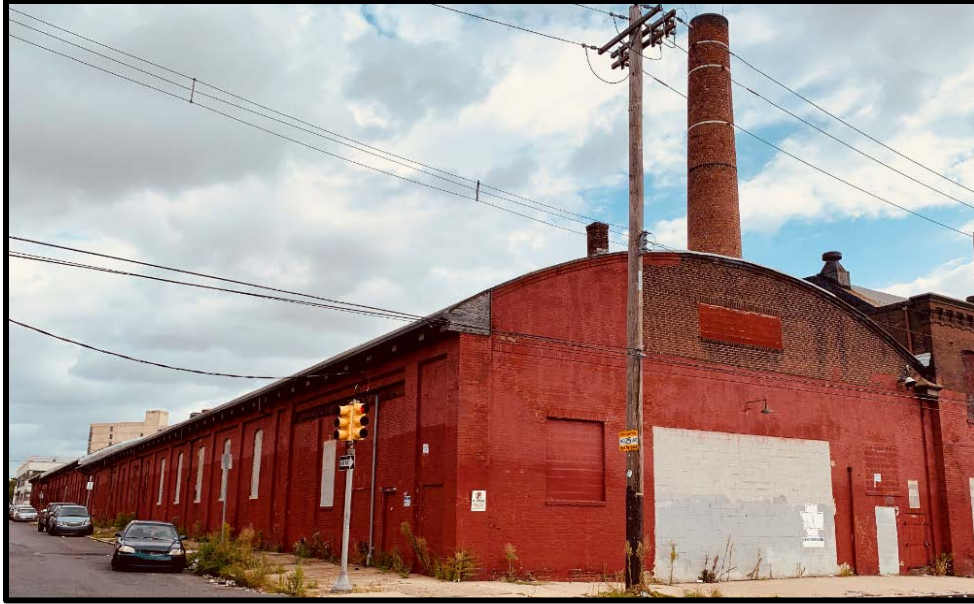
Figure 9. The west and south elevations of Building 2. Source: Oscar Beisert, 2019.
