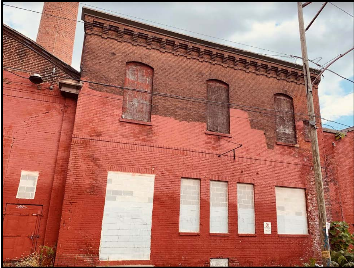
Figure 8. The south elevation of Building 1. Source: Oscar Beisert, 2019.
