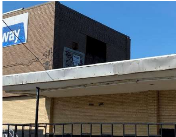
(Photo #3.4) Missing Coping Stones
