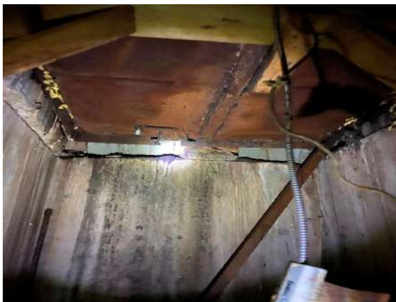
(Photo #7.1) Deteriorated Sidewalk Hatch Frame
