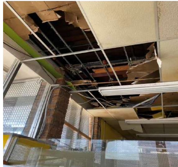
(Photo #1.4) Water Damaged Ceiling Tiles
