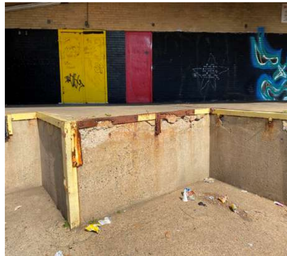
(Photo #4.4) Concrete Spall and Rusty Steel
