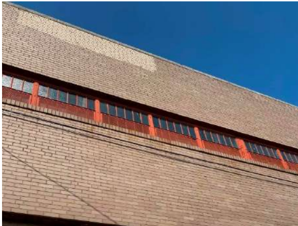
(Photo #3.3) Overhanging Brick on Lintel
