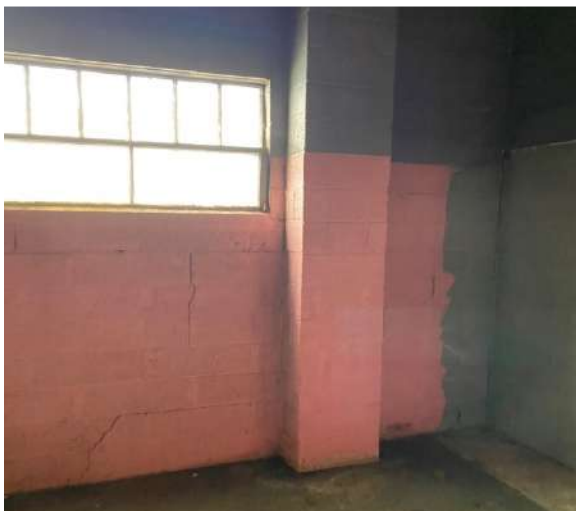
(Photo #3.5) Wall Cracks at Second Floor
