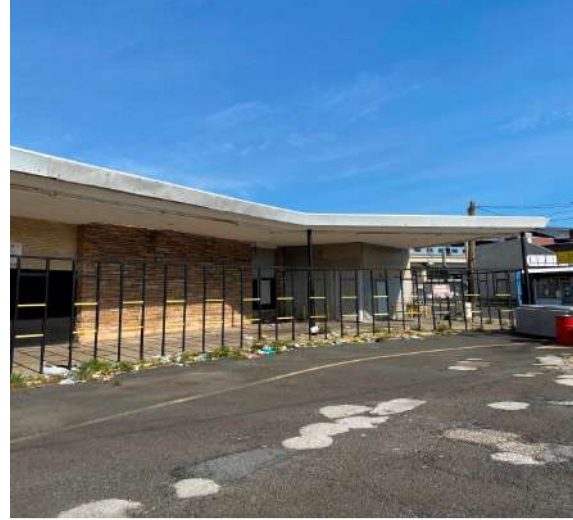
(Photo #1.2) Pitch in Canopy Framing
