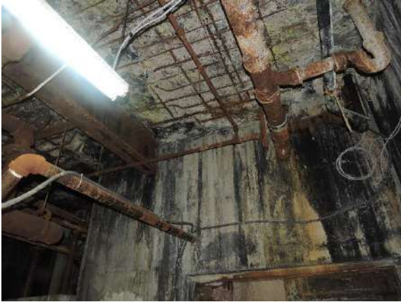
Figure 3: First floor slab over the basement utility room
