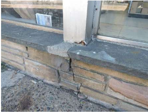
Figure 4: Expansion of the steel has cracked the stone base wall
