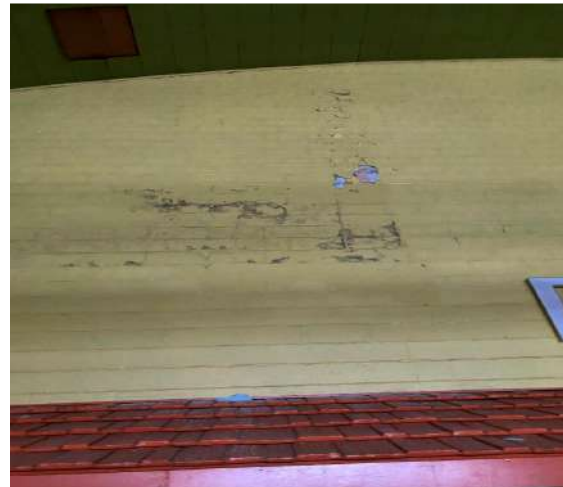
(Photo #2.4) Cracks & Water Damage End Wall
