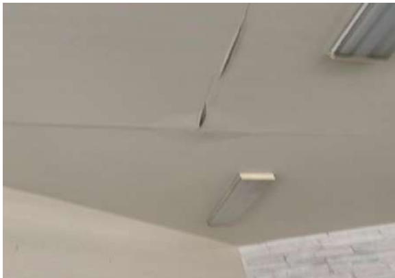
(Photo #6.1) Water Damage in Ceiling
