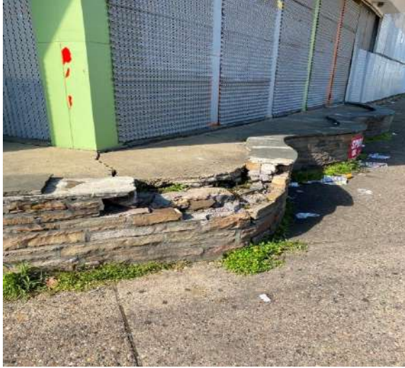
(Photo #1.1) Cracks in Stone Wall Base
