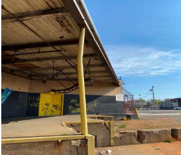
(Photo #4.5) Bent Steel Column
