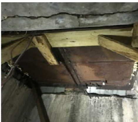
(Photo #3.11) Crack in First Floor Beam
