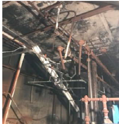
(Photo #3.10) Spall in Underside of First Floor
