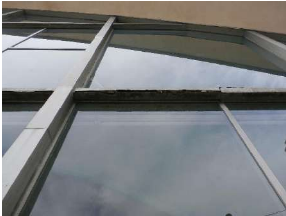
Figure 3: Detail at corroded steel, which cracked the upper glass pane at its lower left corner
