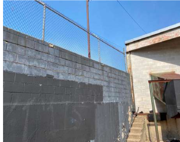
(Photo #4.2) Deteriorated Joints in Retaining Wall
